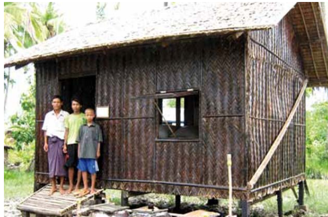
Figure 14: Shelter built using locally available materials including toddy palm and bamboo. (Shelter Projects, 2010, p.63)
