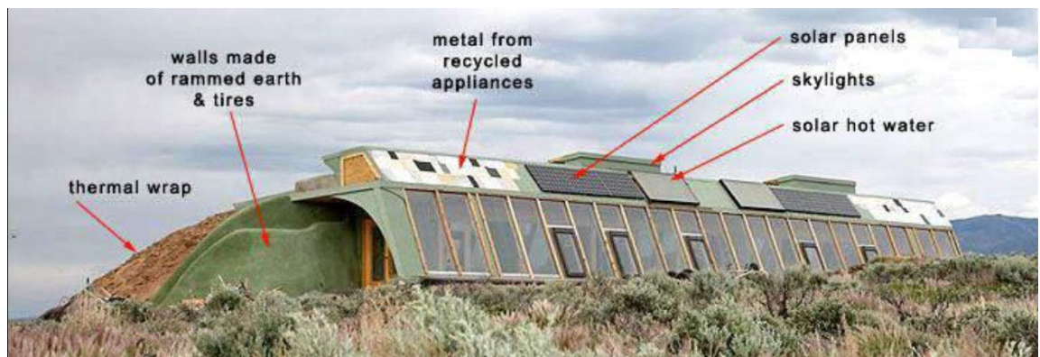
Figure 22. The Earthship as a sustainable home, which is designed to integrate with nature as an example of biomimicry in the Ecosystem level (Anous, 2015)
