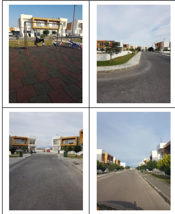
Figure 59: General view of common spaces
