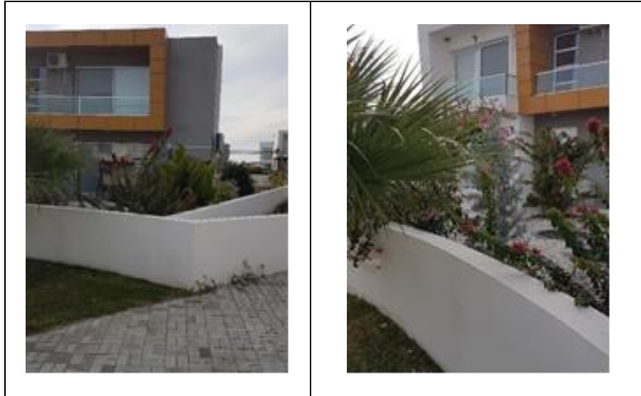
Figure 33: Colours used on the facades of the buildings and coating materials.
