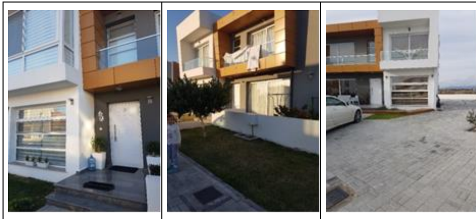
Figure 39: Balconies on the first floor.
