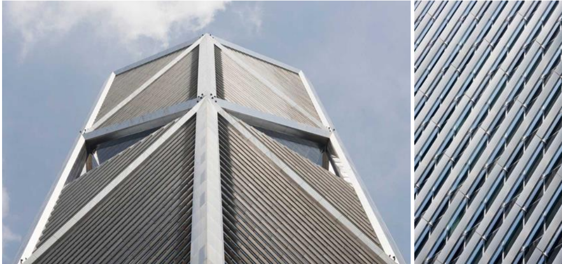
Figure 20: Utilization of Shading and Opaque Frit on High Performance Glazing to Reduce Glare and Solar Heat Gain (Ha, 2013).
