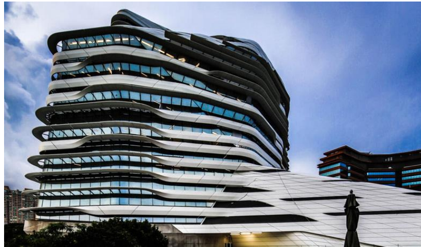
Figure 45: A render of the covering layer which used as shading design of JCIT Source: http://www.arch2o.com
