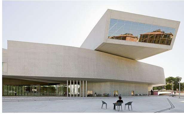
Figure 49: general view showing the different levels and layering technique in Maxxi Museum project Source: Hadid, 2009
