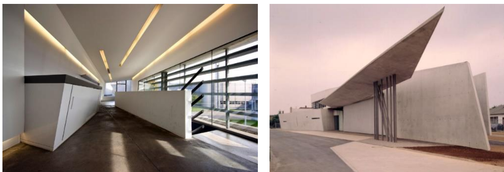
Figure 58: the strong relationship between the exterior and interior of Vitra fire station. Source: https://deavita.com/
