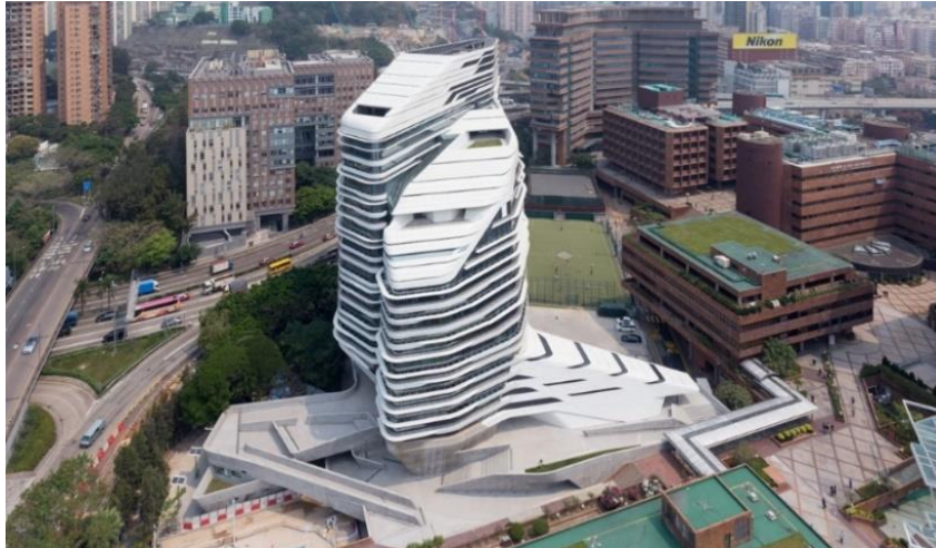
Figure 48: Bird eye view of Jockey Club innovation tower Source: http://worldarchitecture.org
