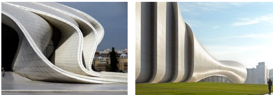
Figure 29: layered curved volumes are clad in pristine, white tiles in Heydar Aliyev Museum Source: http://www.zaha-hadid.com
