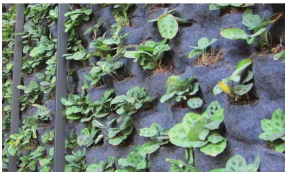
Figure 8: An example of a hanging pocket living wall system (Irina Susorova, 2013)
