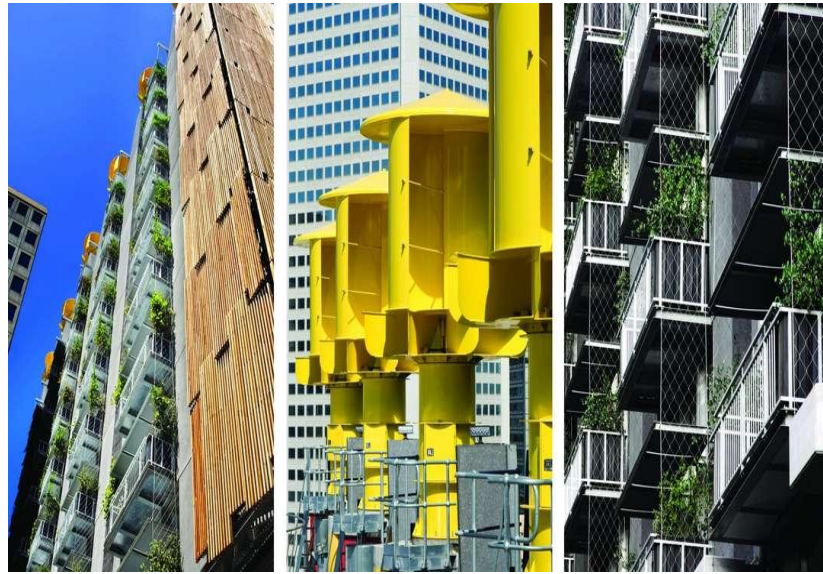
Figure 59: View of CH2 Council House 2 Melbourne, Australia (Dianna Snap, 2013)
