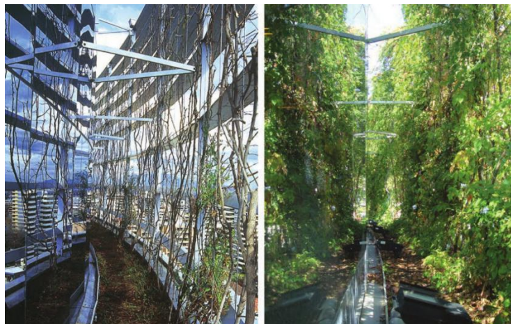
Figure 54: Detailed view of the planter and grid support system, the left image shows the system in winter, when plants are bare, allowing solar penetration into the building.
