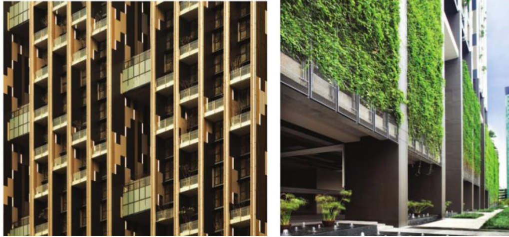
Figure 46. Detail view of façade and climbing plants at exterior of podium car park showing the overhangs and deep vertical fins.
