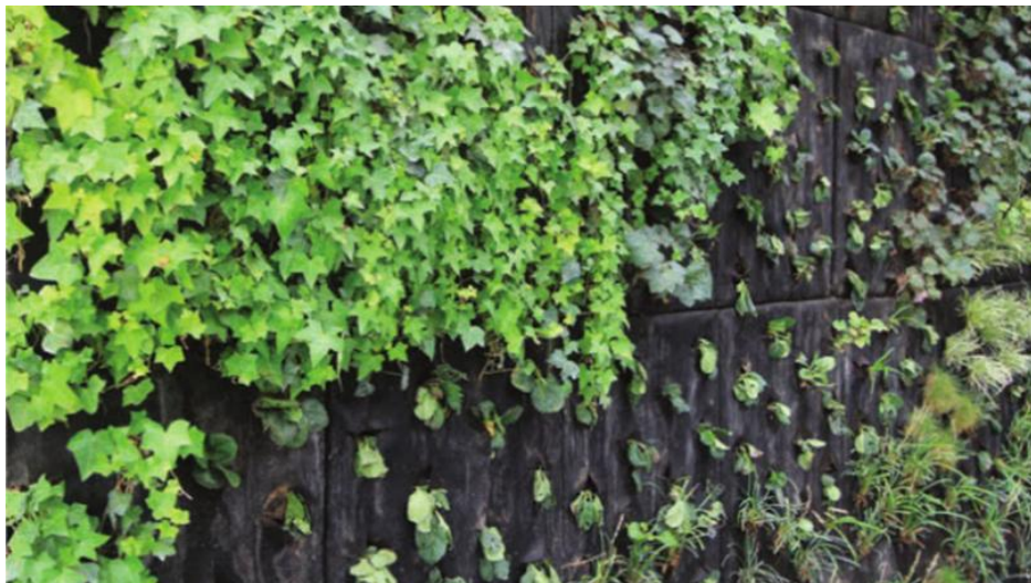
Figure 6: An example of a vegetated mat living wall system (Irina Susorova, 2013)
