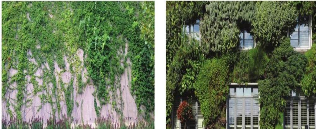
Figure 1: Example of façade-supported green wall (left) and living wall (right) (Irina Susorova,2013)
