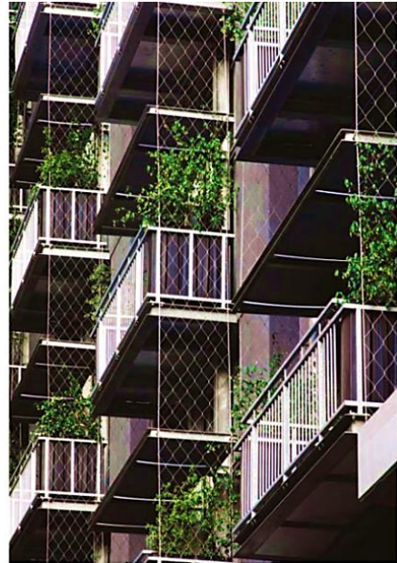
Figure 61: Conceptual diagram highlighting the importance of daylight shading at the north side and climbing plants growing onto metal mesh screens on north façade (Author, 2016)
