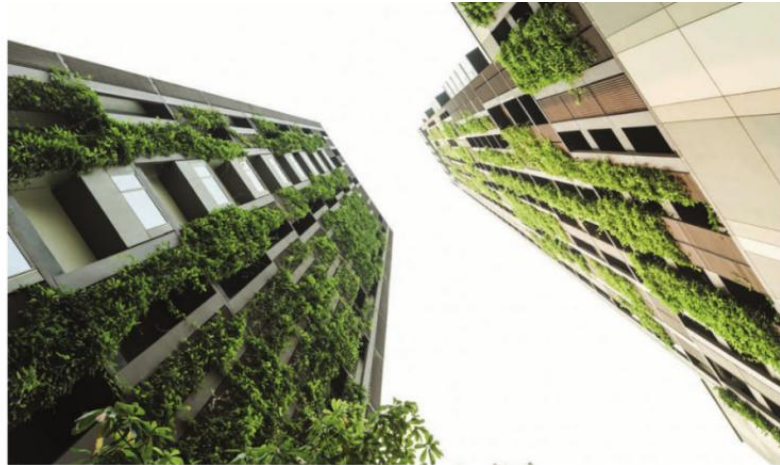
Figure 40: View of green walls between the buildings
