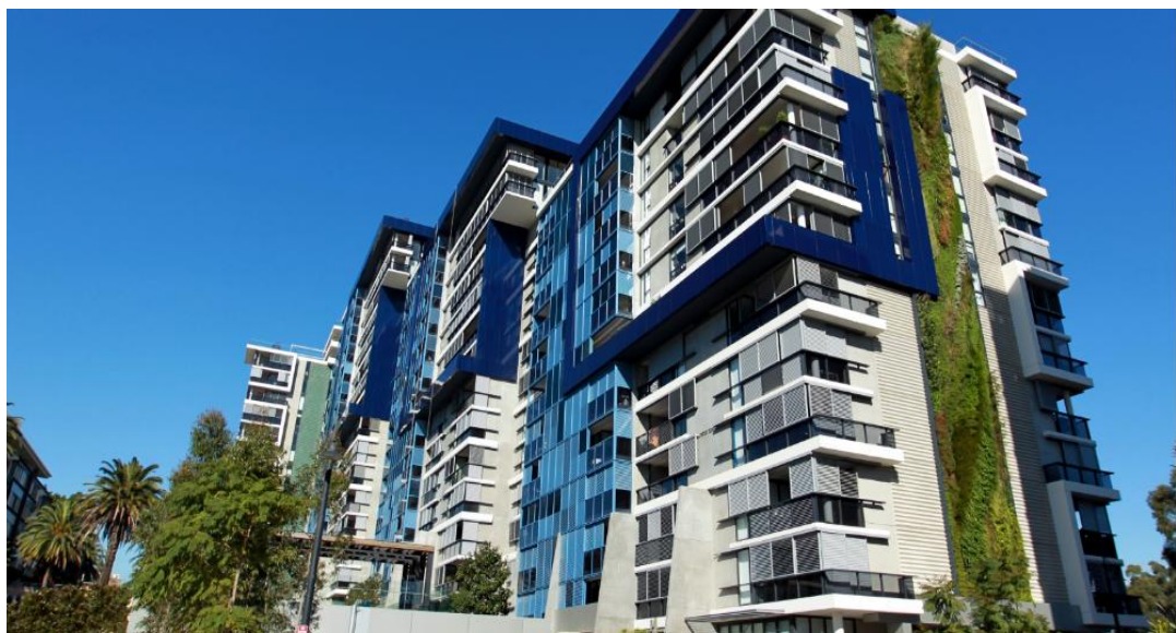
Figure 29: North view of building, a combination of cladding material, concrete, and green wall (Fender Katsalidis, 2011)
