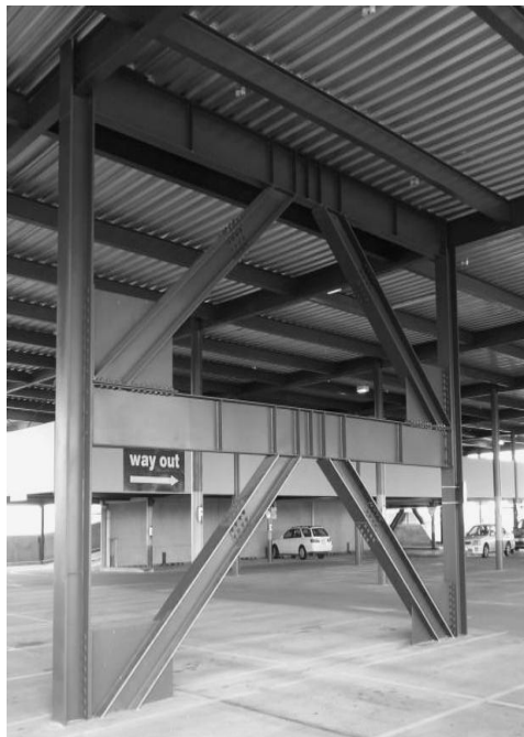
Figure 1.4: Eccentrically braced frames in practice ( www.civilweb.ir )
