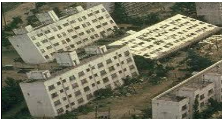
Figure 3.5: Loss of property due to liquefaction (USA Geological Survey)
