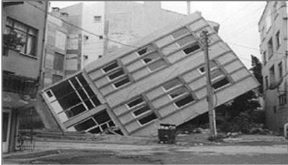
Figure 3.4: Destruction in buildings as a result of liquefaction (Madabhushi, 2007)
