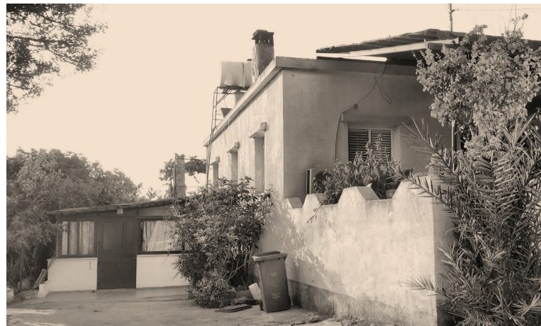
Figure 4.11: Additional kitchen and the storage build outdoors. (Taken by author)
