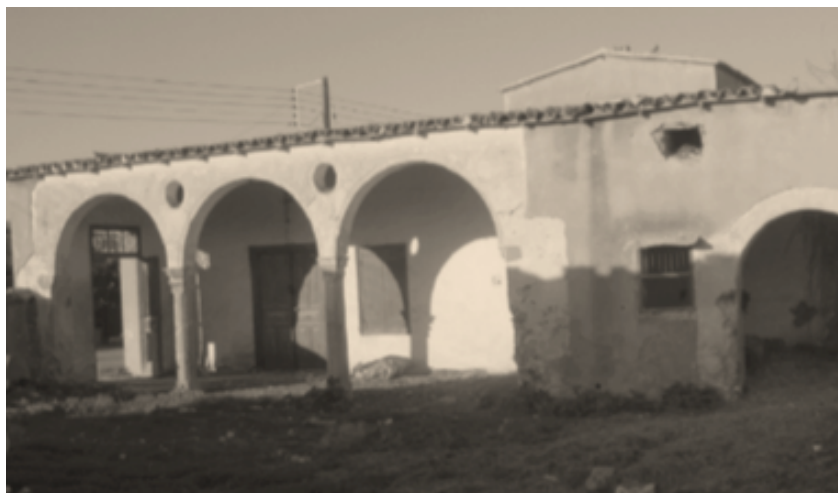
Figure 3.4: The unique arcaded house form of the traditional Cypriot settlements. (Dinçyürek and Türker, 2006)
