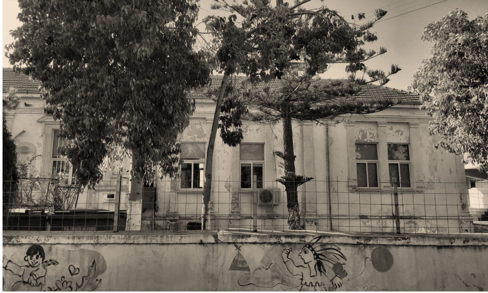
Figure 2.11: Elementary school building in Yeni Erenköy. It is still being used as an elementary school with the additional buildings (Taken by author).
