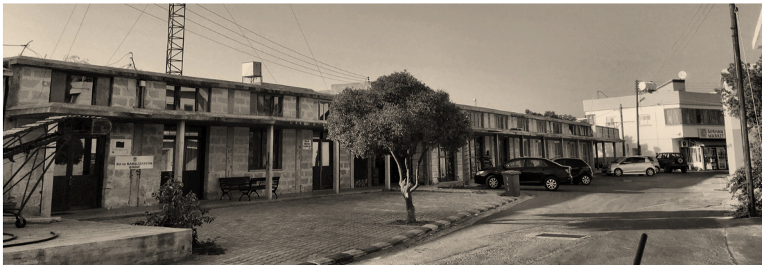
Figure 2.15: Cooperative building in Yeni Erenköy. Currently, some parts of it are leased as a shop (Taken by author).
