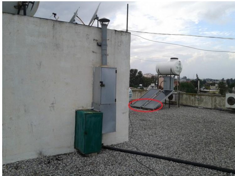
Figure 40. The effect of shading on solar collector energy performance by studying case examples
