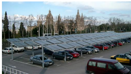
Figure 19. Solar hot water collectors place above parking area ( http://www.yourhome.gov.au/energy/hot-water-service )
