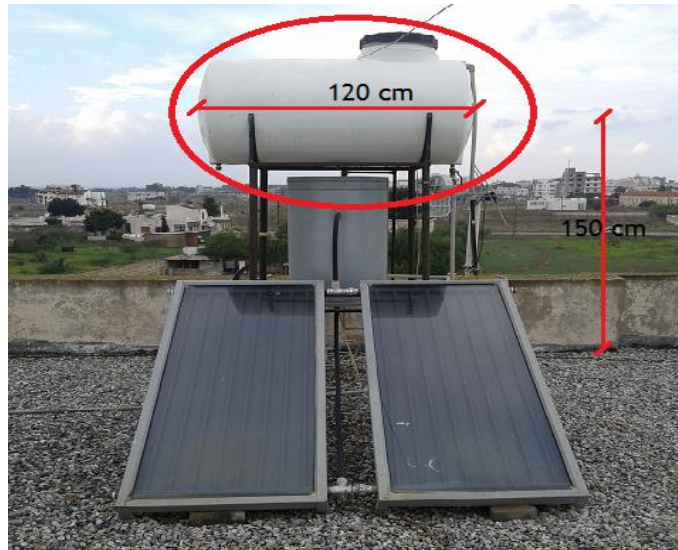
Figure 42. The Water Tank
