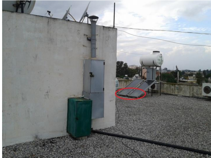
Figure 47. The effects of shading on solar collector's energy performance by roof access
