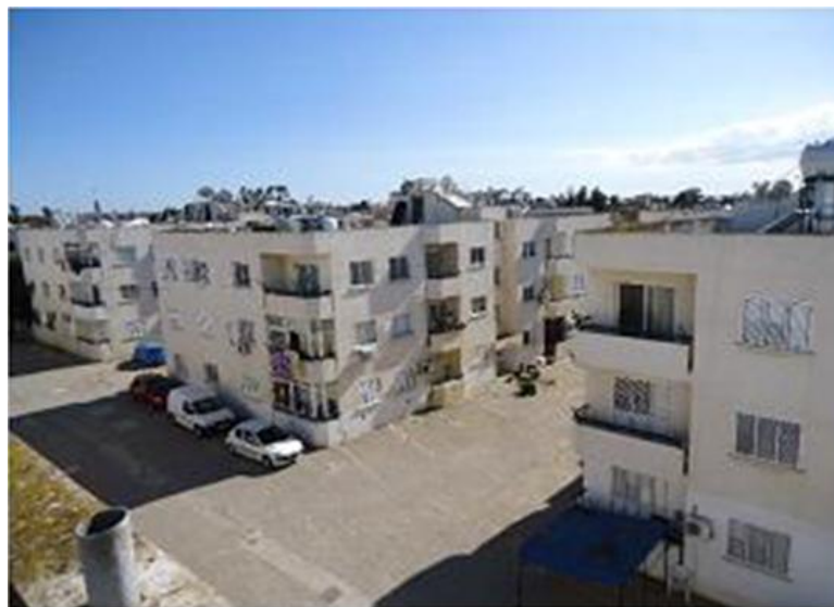
Figure 29. View of Haci Ali Multi-Story Building
