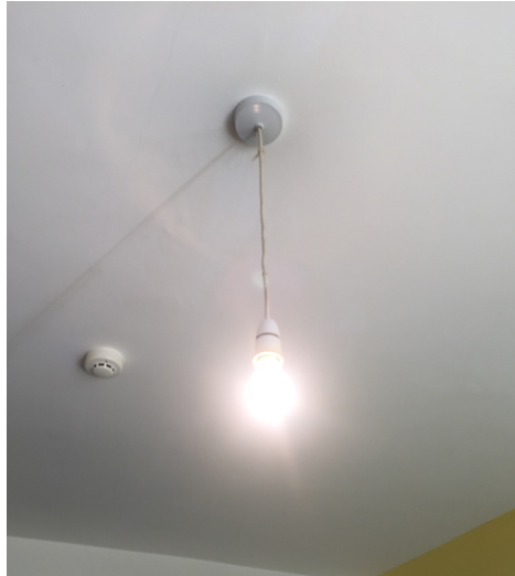
Figure 30: most of the lights are regular incandescent lamps. (Photo taken by author).
