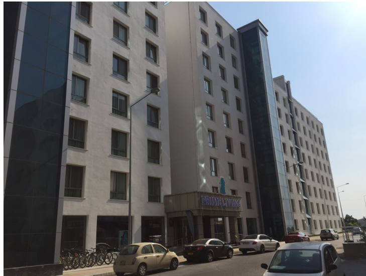
Figure 32: Prime Living dormitory (Photo taken by author).
