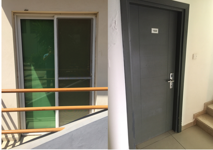
Figure 28: Door and window types in Kamacioğlu dormitory. (Photo taken by author).
