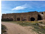
Stone pointed arches + multiple arches with stone posts
