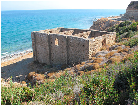
Figure 1. Carob Warehouse in Esentepe village (Photo by Beser Oktay Vehbi).
