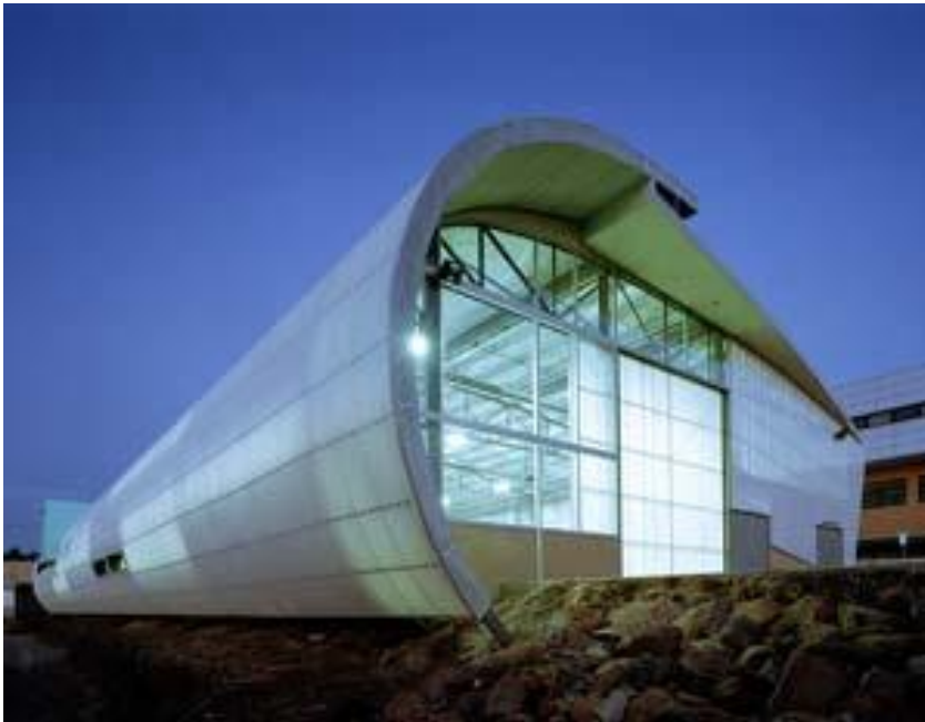
Figure 6. Polymer Engineering Center, Cox Sanderson Ness, Victoria, Australia. (Boschetti, 2002: 62)
