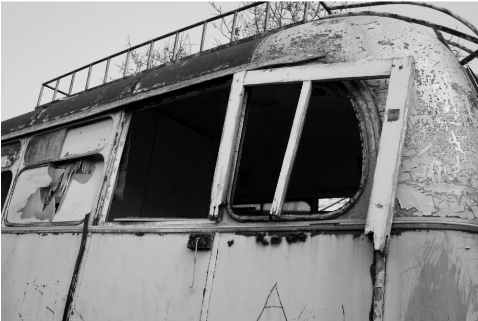
Figure 6. Remains of a hand-made shutter on the west facade of the bus-house.
