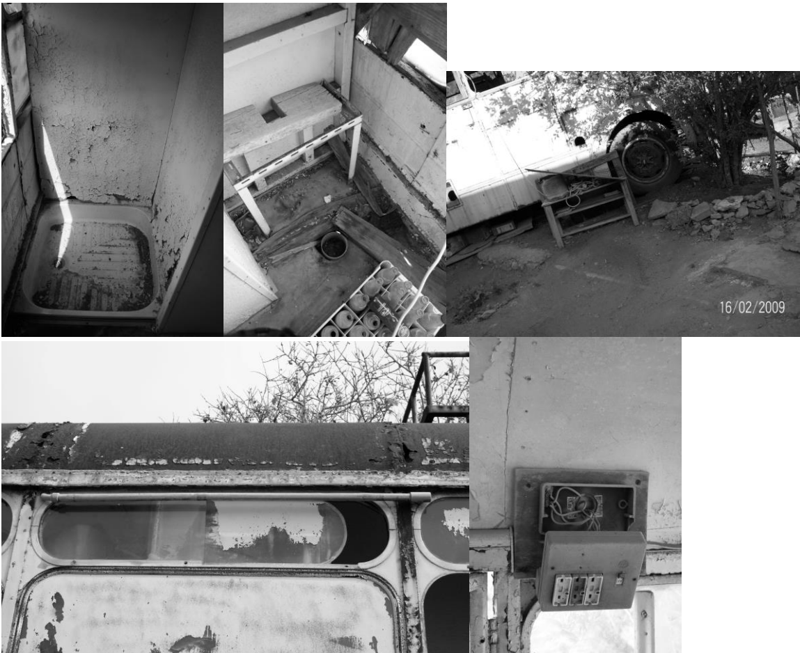
Figure 4. Service systems of the bus-house. (a.bath tube, b.place of toilet, c.sewage connection, d.water supply, e. electric fuses)
