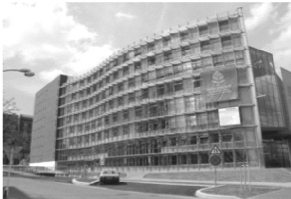
Figure 22: Solar Double Ventilated Facade on the Southern Wing of Brno Moravian Library (Jaros et al., 2002).
