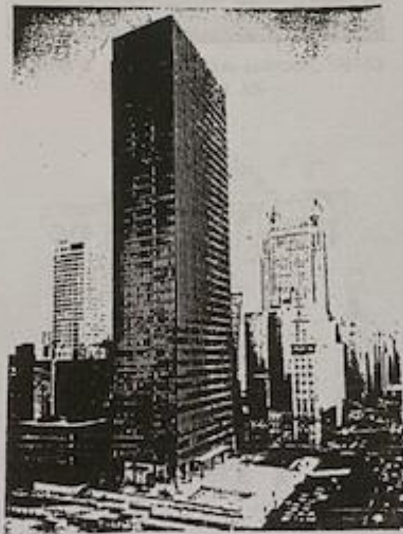
Figure 1. Seagram Building, NY, 1958 Source: Stern, R.A.M., Modern Classicism, Thames and Hudson Ltd., London, 1988, p.31
