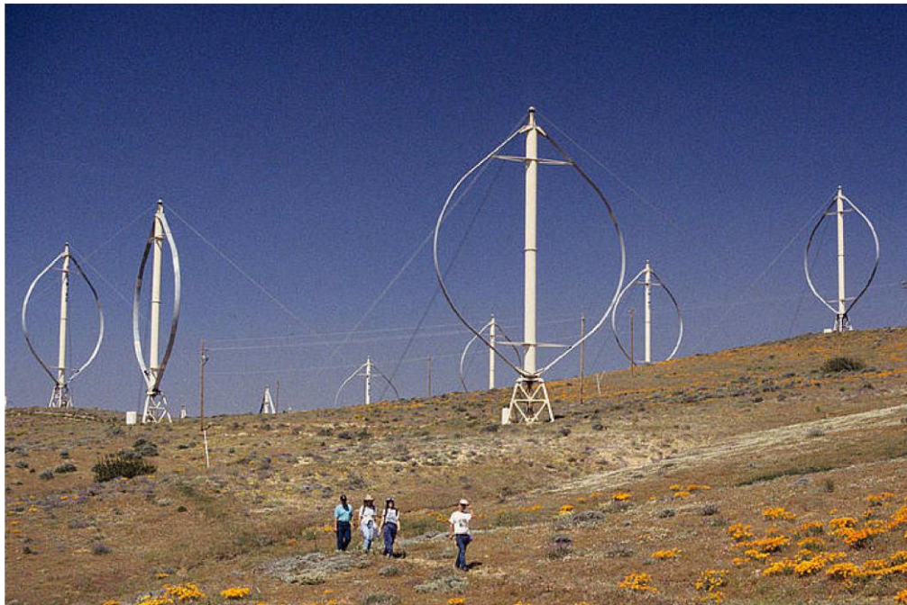
Figure 13 : FloWind Turbine along the Tehachapi Pass [21]
