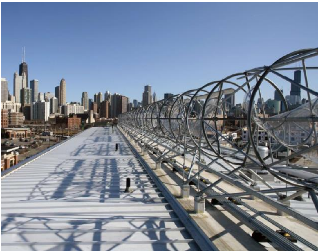
Figure 17 : Aerotecture turbines on Mercy Housing Lakefront rooftop –Chicago [25]
