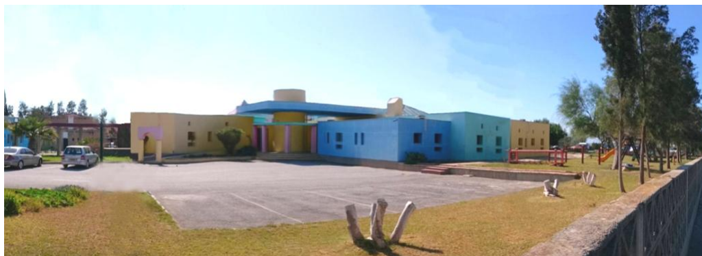
Figure 58: The simplifying in the building design as a modular concept increases the legibility of the space for children - S.O.S Kindergarten (Direct Observation on 22/02/2016)
