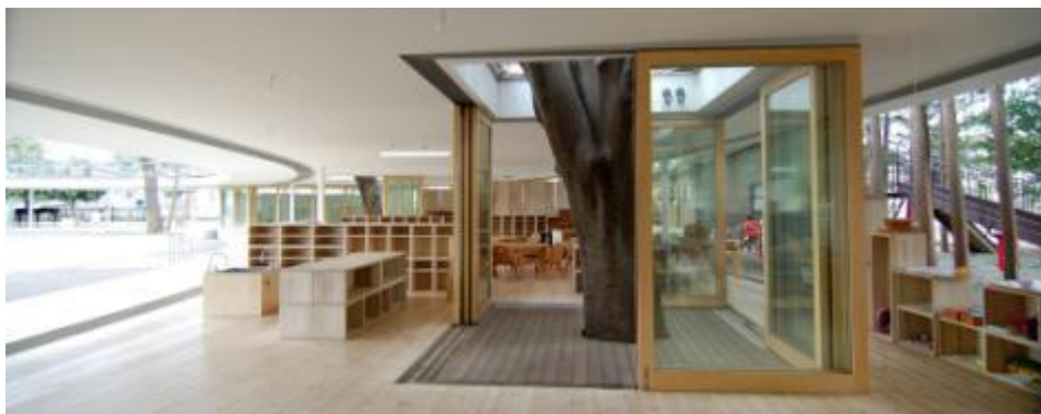
Figure 24: Fuji kindergarten – Completely open planning inside the building, without any fixed Wall
