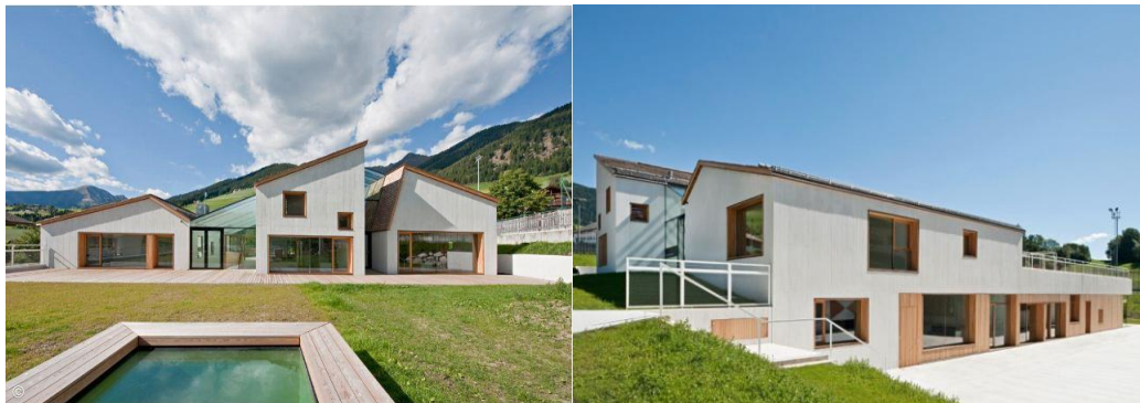
Figure 32: Kindergarten Terenten – Three Houses
