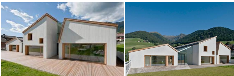
Figure 33: Kindergarten Terenten – Three Houses
