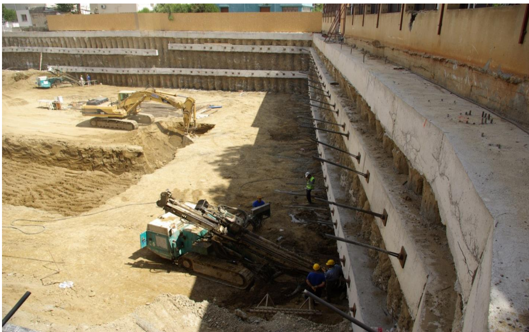
Figure 9.13: Anchorage in stage 3
