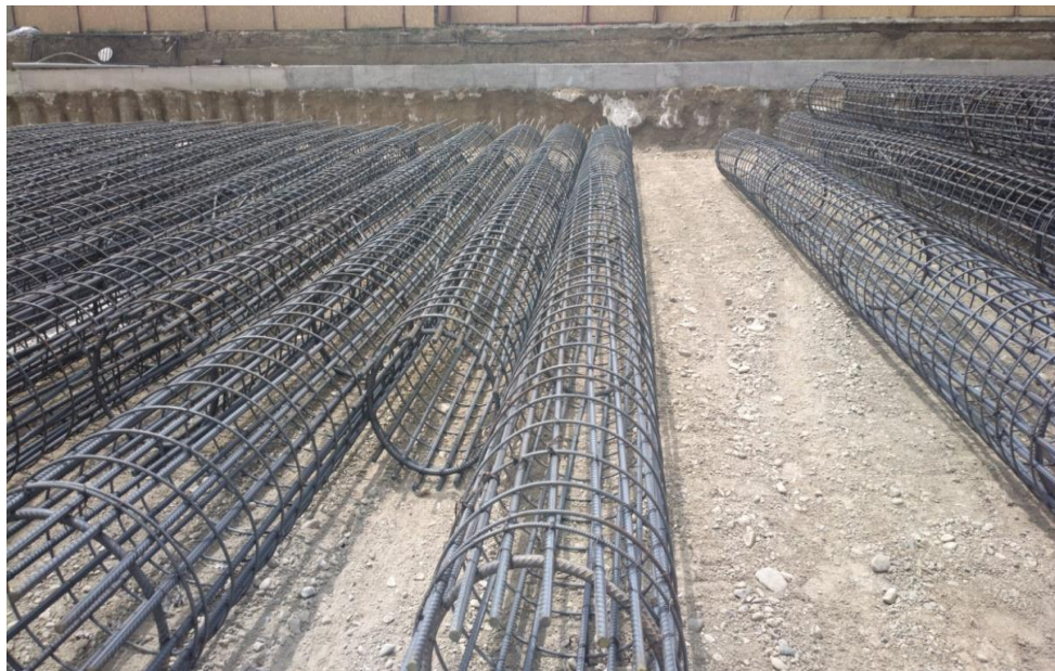
Figure 9.11: Steel cages for piles of wall
