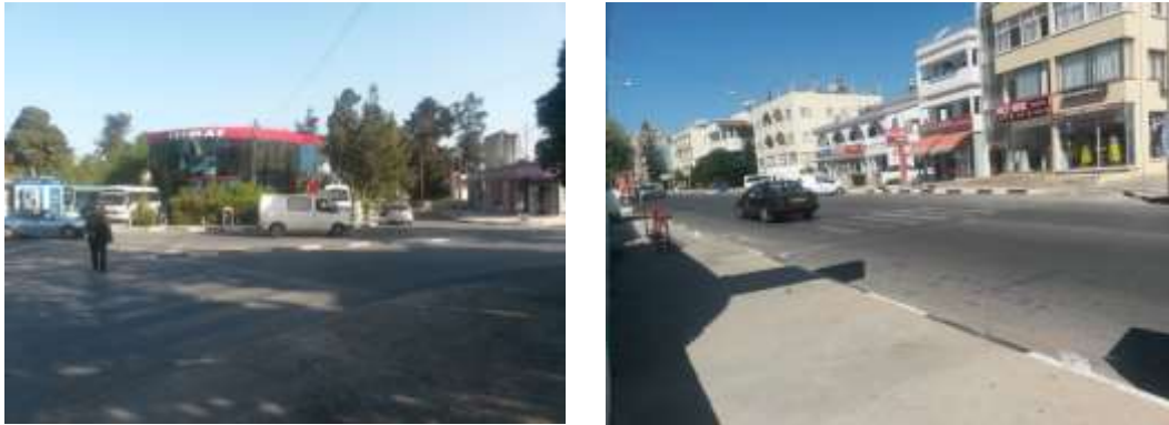
Figure 51: Lack of any signs to aware crosswalker and drivers
