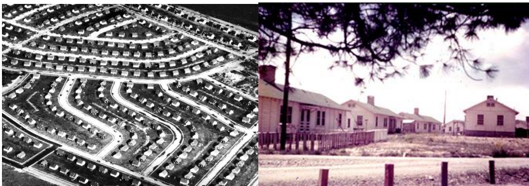
Figure 35: Mass production of ranch houses after World War 2 (Prown, 1982).
