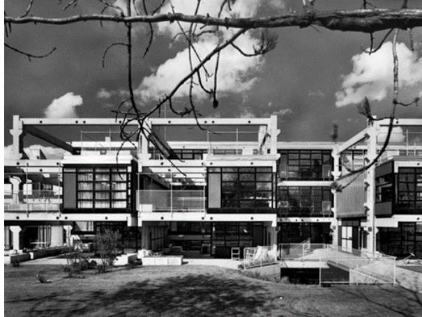
Figure 46: Genter Strasse Building, Munich in 1972 (Schneider&Till,2005).
