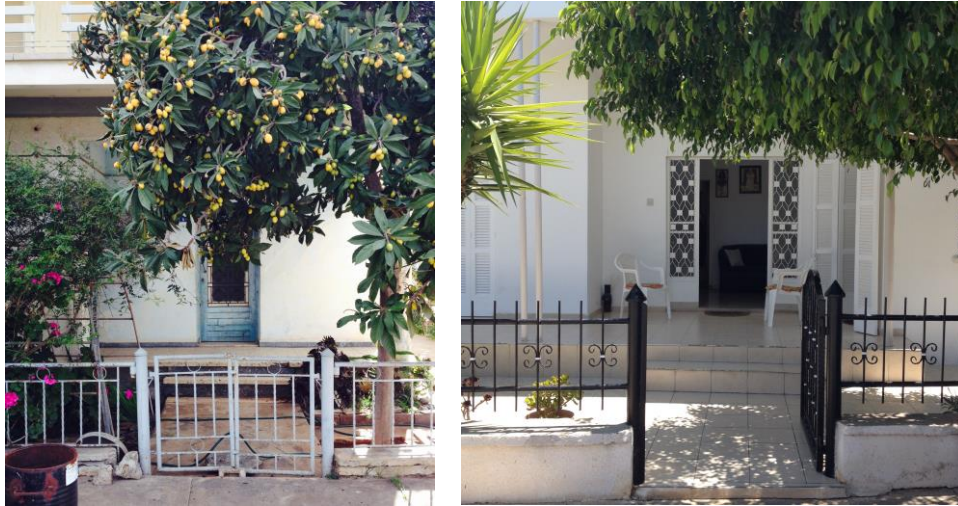
Figure 12: Entrance view of Aşağı Maraş Homes (Taken by the author)
