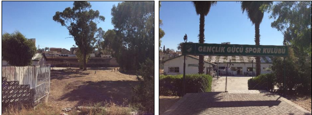
Figure 3.57: Neglected environment and inactive building at the Zone 6
