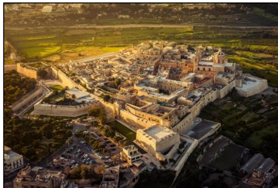
Figure 2.12: Walled City of Mdina, Aerial View, Malta. URL,9
