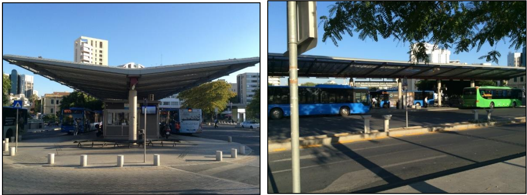
Figure 3.88: Images from Solomos square and Bus Station area
