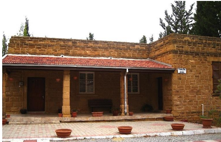
Figure 4.3 One of the two identical classroom blocks of Teachers Training College.
