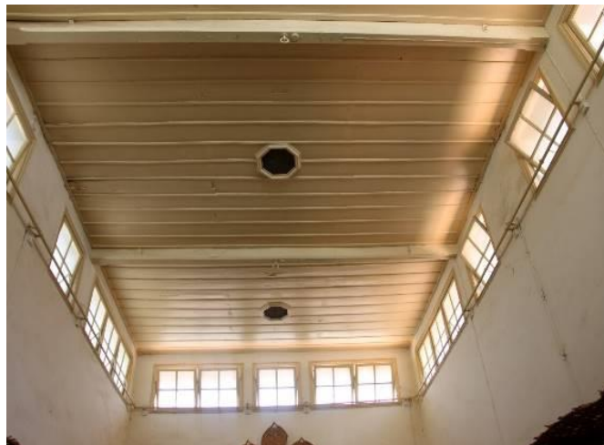
Figure 3.2. A view of the roof from Idadi's interior.
