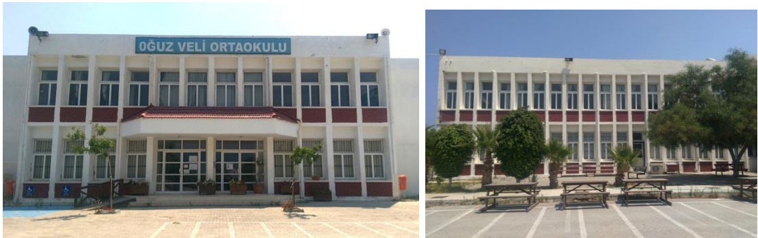
Figure 6.5. Front and left side (West) views of Oğuz Veli Secondary School, Kyrenia.
