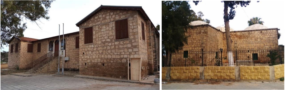
Figure 5.4. Front and back views of Kutup Osman Complex.
