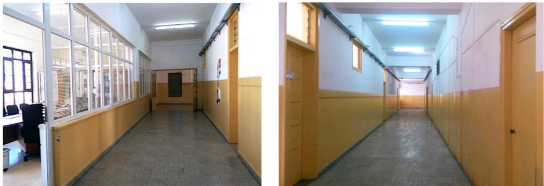
Figure 5.2. Views from the corridors. On the left the administrative office, on the right classrooms and workshop areas.
