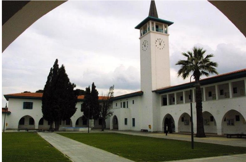
Figure 6.3. Nicosia Teachers' Training College (Source: Cyprus Mail , 27 October 2010). The building is one of the most representative public buildings belonging to the British mélange policy.
