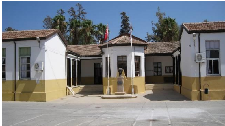
Figure 3.5. Front and back view of Gazi Elementary School.
