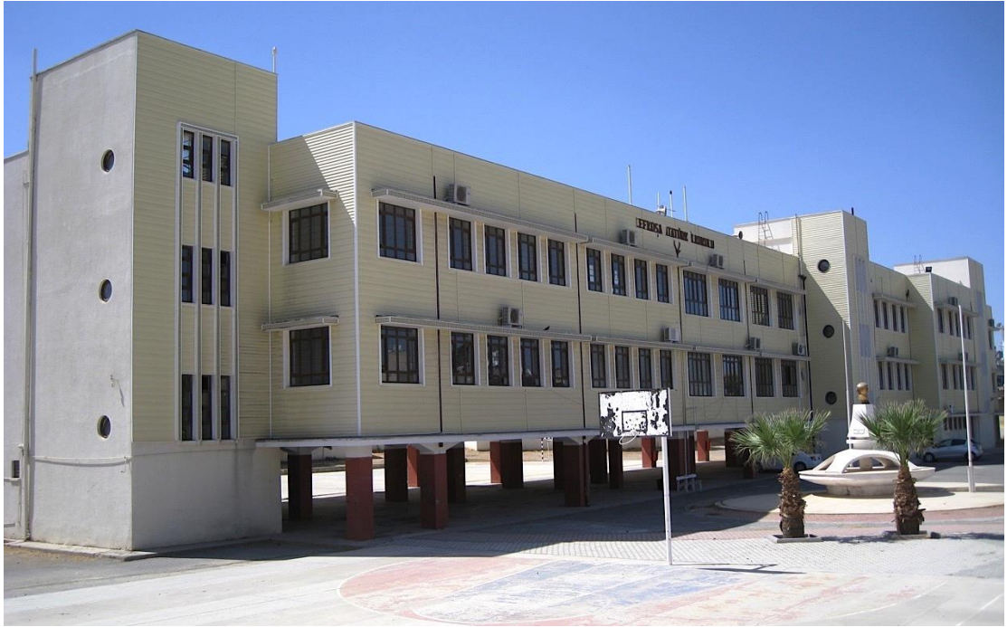
Figure 5.1. A view of Atatürk Elementary School with recent cladding.
