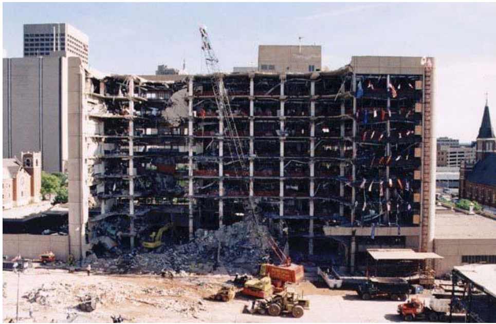
Figure 2.2: Alfred P. Murrah Federal building (FEMA-427, 2003).
