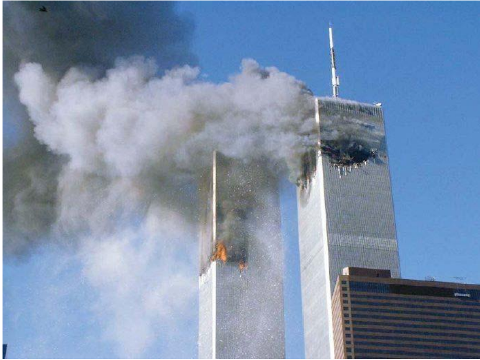
Figure 2.3: World Trade Center twin towers after the terrorist attack (FEMA-403, 2002).
