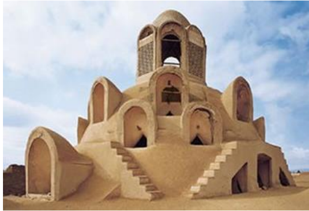
Figure 23. Mud as a main material in shaping construction process of Iranian traditional houses (Reference: URL 9).
