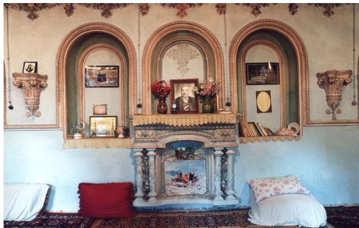
Figure 18. Design Niche in a specific height to be reachable while people sitting or standing (reference: URL 5).
