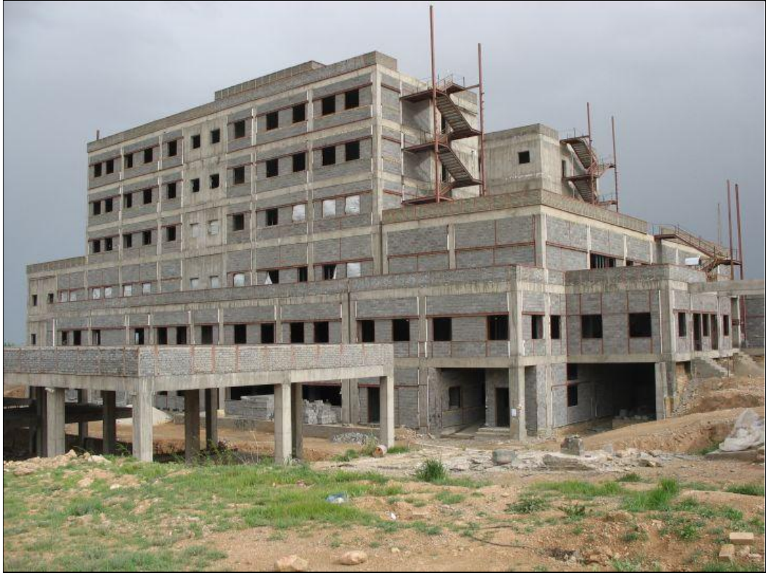
Figure 8: Abhar hospital – case study 9
