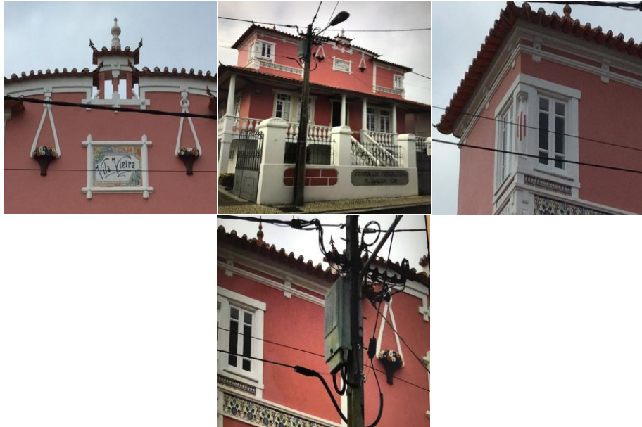
Figure 5.44: The preservation of Villa Vieira Photo by Shahrbanoo Nov, 20
