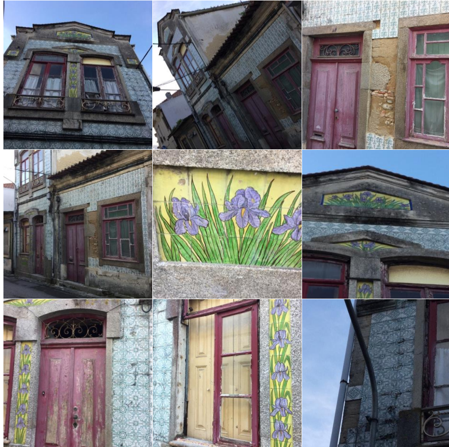
Figure 5.35: The preservation of Edificio dos Lirios Photo by Shahrbanoo Jun, 2017
