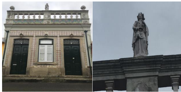
Figure 4.58: R. Marechal Zagalo, 59 Photo by Shahrbanoo Jan 2017
