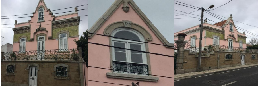
Figure 5.39: The preservation of building No 19, Rvasco da Gama Photo by Shahrbanoo Nov, 2017
