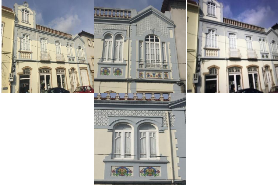
Figure 5.47: The preservation of building No 40, Rvasco da Gama Avenida Vsconde de Salreu, Starreja Photo by Shahrbanoo Nov, 2016
