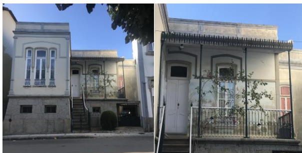
Figure 4.42: Chalet of the Vidal family in Albergaria-A-Velha Photo by Shahrbanoo 5 Nov 2017
