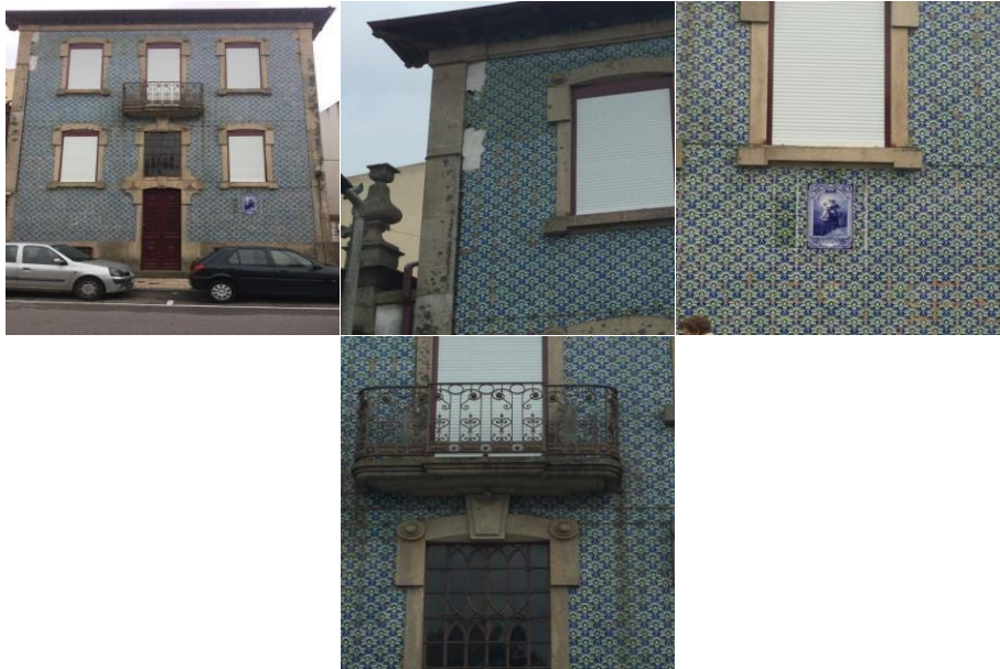
Figure 5.51: The preservation of building No 54, R. Candido dos Reis,Ovar Photo by Shahrbanoo, Dec,2016
