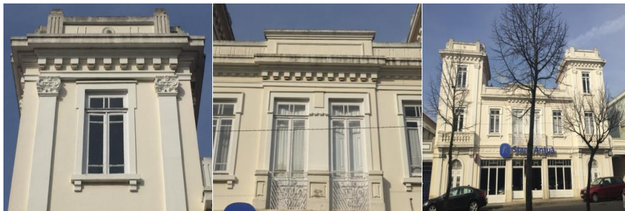
Figure 5.50: The preservation of building No 43, Rvasco da Gama Avenida Vsconde de Salreu, Starreja Photo by Shahrbanoo Nov, 2016
