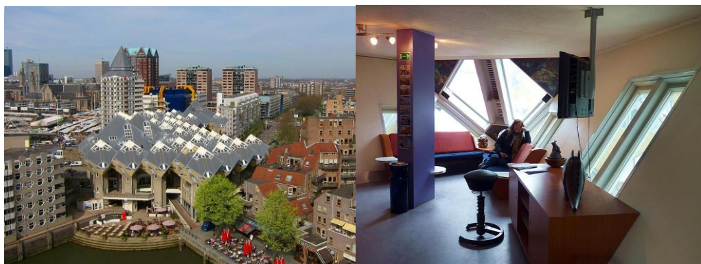
Figure 12. Cube houses in Rotterdam, an iconic building with unconventional typology designed by Piet Blom in 1984, has been renewed and converted into a new Stayokay hostel (taken from Türkan Uraz archives, 2016)
