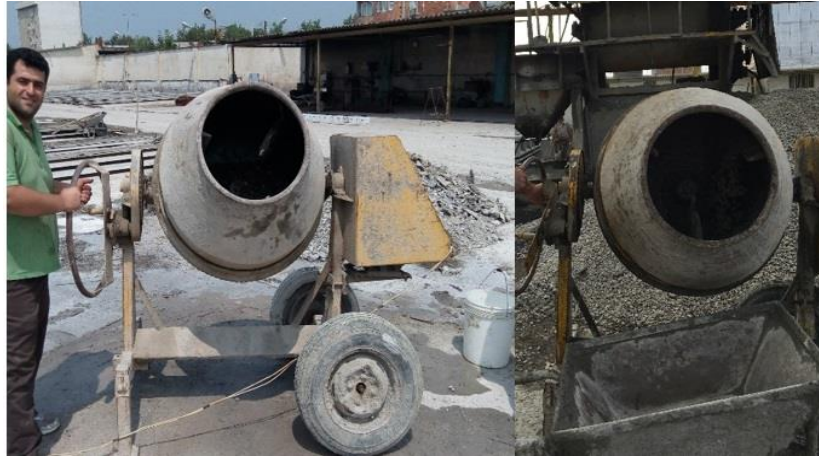
Figure 3.3: Mixing of the materials for build the concrete by mixer
