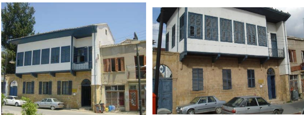
Figure 3.6: The main façade of Dervish Pasha Mansion (Author, 2015).
