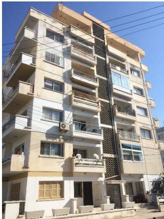
Figure 15. Single Apartment Building (Akmanlar2), Magusa (Author,2018)
