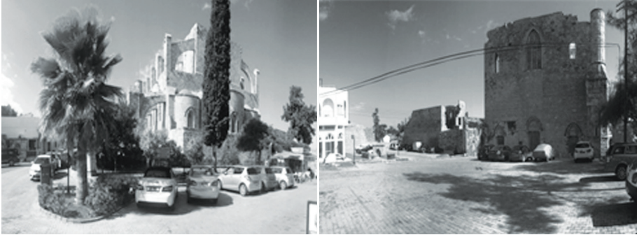
Fig.9 (Left) East & South Facade of the St. Peter & Paul Cathedral, Constant vehicular movement and parking, blocks the contact zones and most frequent pedestrian axis (source: author)
