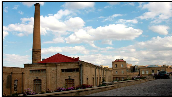
Figure 28. General view from Khosravi leather complex after conservation
