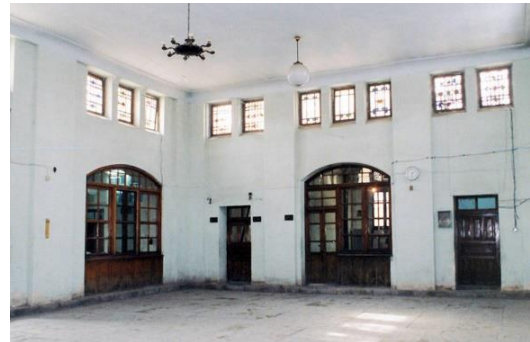
Figure 58. Office building (Ghasemi, 2017)
