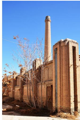
Figure 80. The cooling tower
