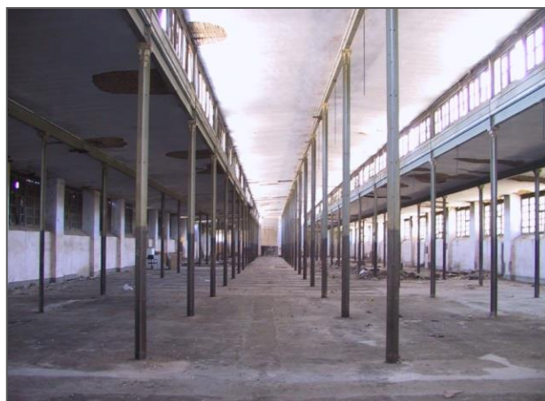
Figure 64. Metallic porter columns of manufacturing hall (Ghasemi, 2017)
