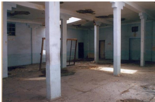
Figure 71. Metallic porter columns and beams (Ghasemi, 2017)
