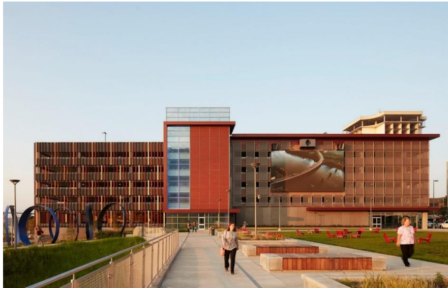
Figure 26. The building with parking spaces (Dezeen, 2019).
