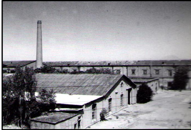
Figure 27. General view from Khosravi leather complex before conservation
