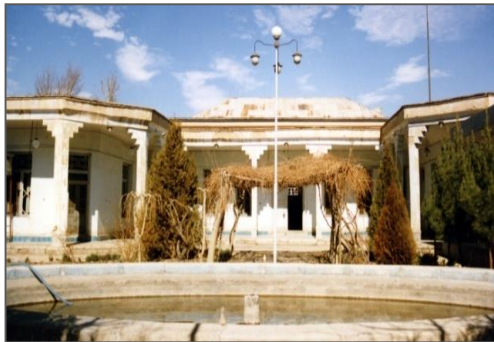
Figure 57. Office building (Ghasemi, 2017)
