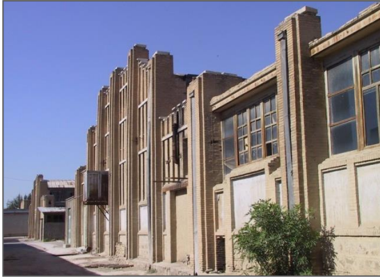
Figure 59. West view of the manufacturing halls (Izadi, 2017)
