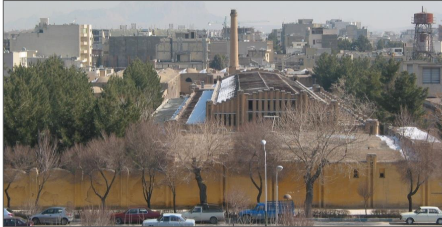
Figure 44. General view of Risbaf factory from Chaharbagh Street (Author)
