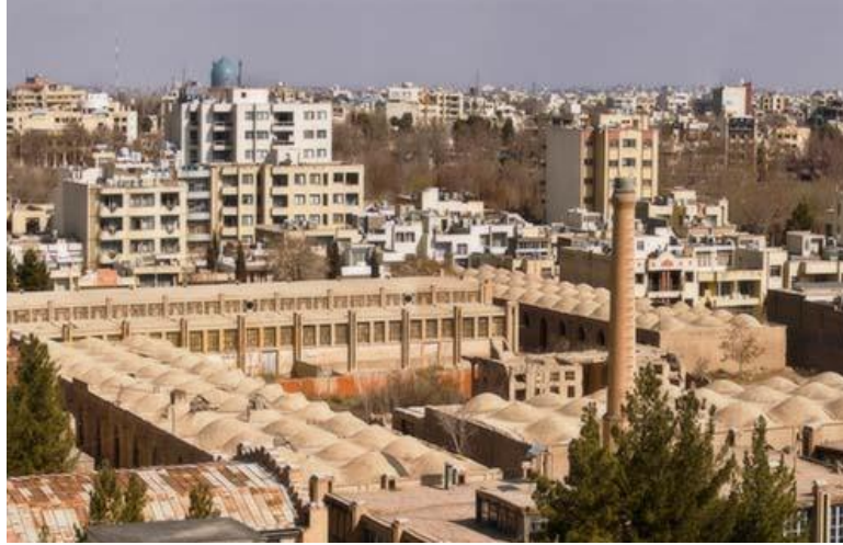
Figure 54. General view of Risbaf factory
