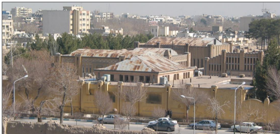
Figure 43. General view of Risbaf factory from Chaharbagh Street (Author)
