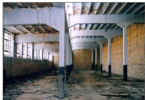
Figure 72. The metal construction of the building (Ghasemi, 2017)
