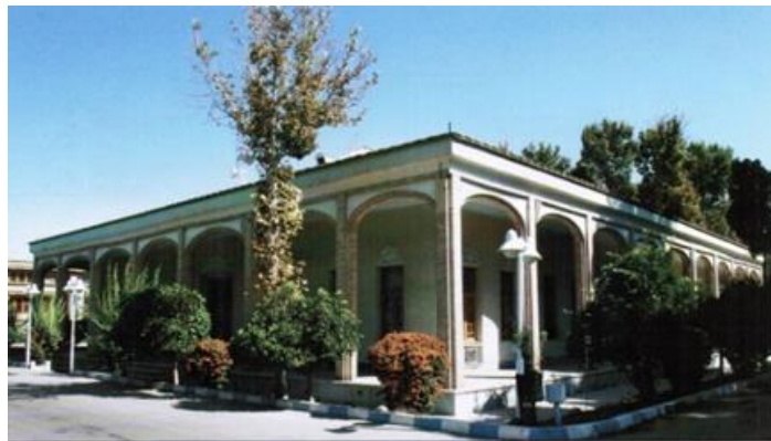
Figure 39. South view from the office building
