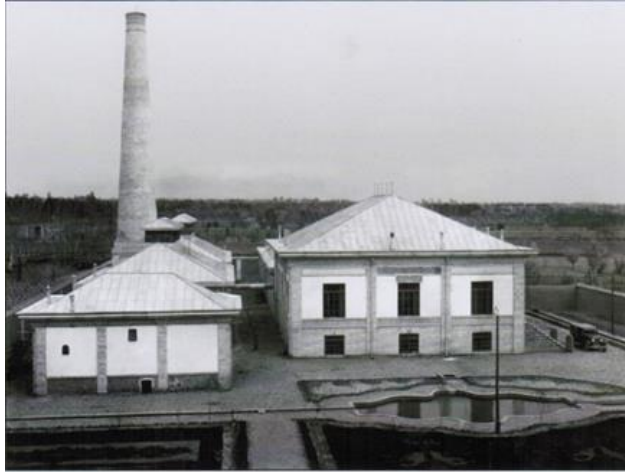
Figure 40. General view from Beryanak factory before conservation (Haft-chenar museum of Tehran archive, 2018)
