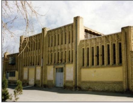
Figure 73. Porter columns with a brick view (Ghasemi, 2017)
