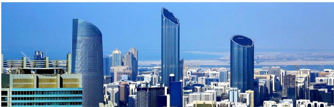
Figure 3.20: Burj Mohammed Bin Rashid
