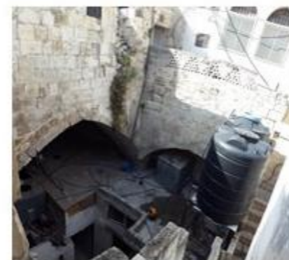
(P6): The opening of the Iwan toward the courtyard
