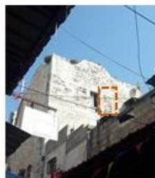
(P1) The openings in west elevation
