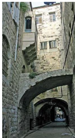
Picture 5: Two types of qantara in the old city of Nablus- the arched one without room and the vaulted zone with room (Captured by author)
