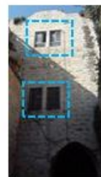
(P1) The openings in south elevation
