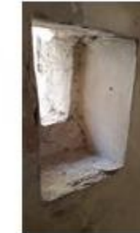
(P2) The details of one small openings toward the street (represent the thickness of the façade)
