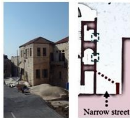
P(12): Openings directed toward the roof of neighbors to prevent any unwanted sight from the house P(12): Section illustrated how the width regulate the line of sight
