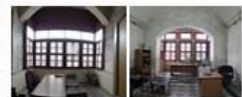
(P11): Meshrabiya openings from the house
