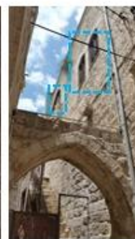
(P6) Exterior south façade
