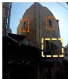
(P1) The openings in east and north elevation
