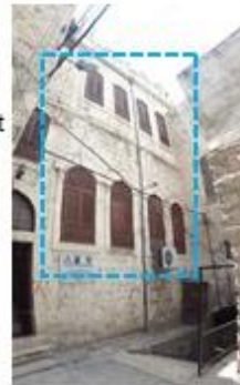
(P1): Openings in the north elevation
