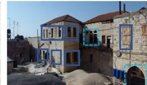
(P4): Openings over the south elevation
