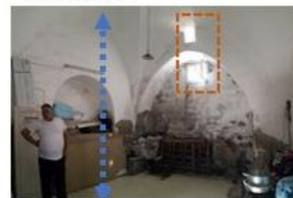
(P1): The location of the opening inside the mansion
