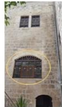
(P3) Wide opening toward the courtyard
