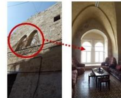
(P4 & 5): The exterior shape smaller than the inside opening to attain visual privacy
