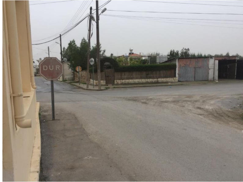
Figure 3.6: Road with Existing Traffic Signs at an Intersection in Geçitkale
