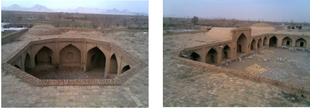
Figure 40. Safavid Black Hole Caravanserai or Sheikh Ali Khan Zanganeh Caravanserai, Shahinshahr and Meymeh City, Isfahan province, Iran (URL32)
