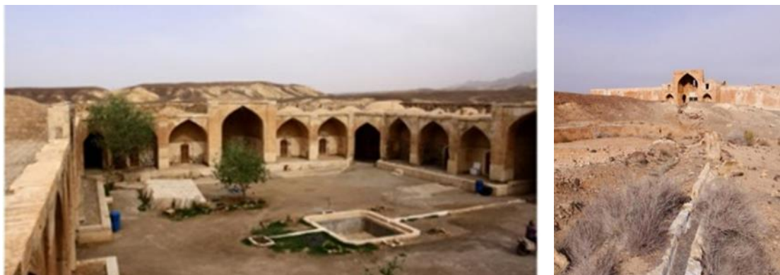
Figure 37. Qasr-e Bahram Caravanserai water supply system, Semnan Province, Iran (URL28)
