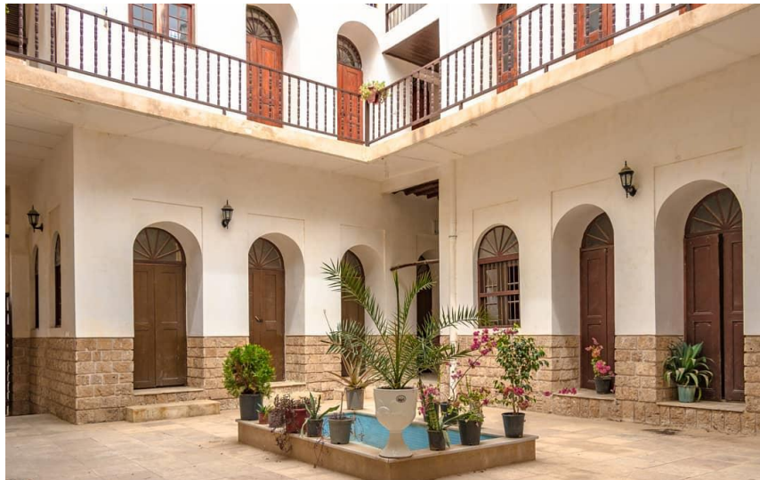
Figure 5.1: Arrangement of openings in the ground and first floor of Rashidy house (M.Saradj 2014)
