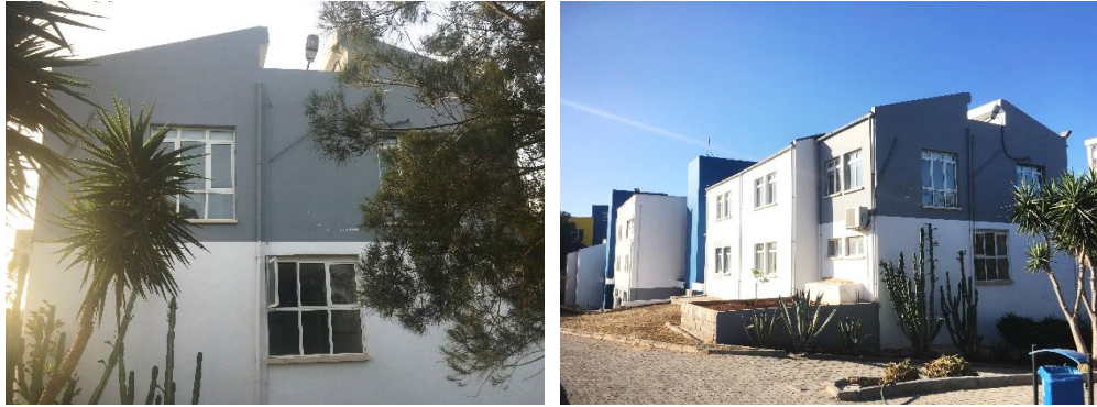
Figure 28: South-East Elevation of the Office Building (Taken by author, 2018)
