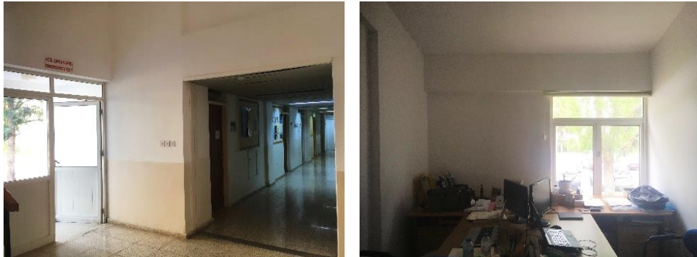
Figure 30: Office and Corridor Located on North-East Side (Taken by author, 2018)
