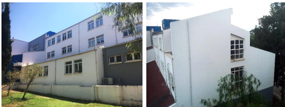
Figure 29: North-East & North-West Elevations of the Office Building (Taken by author, 2018)
