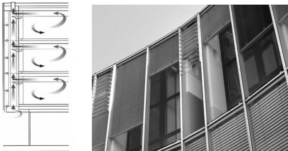
Figure 6: Shaft Box Window Facade (Schulze, Eicker, 2013)
