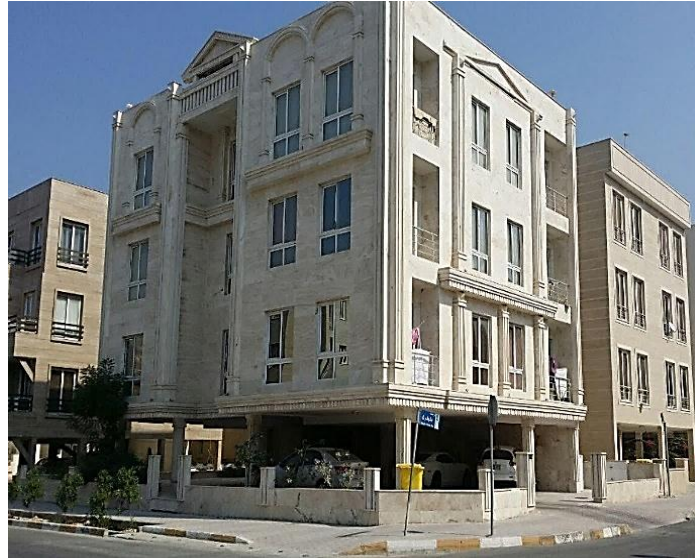
Figure 4.15: Case Study External View (Source: Author)
