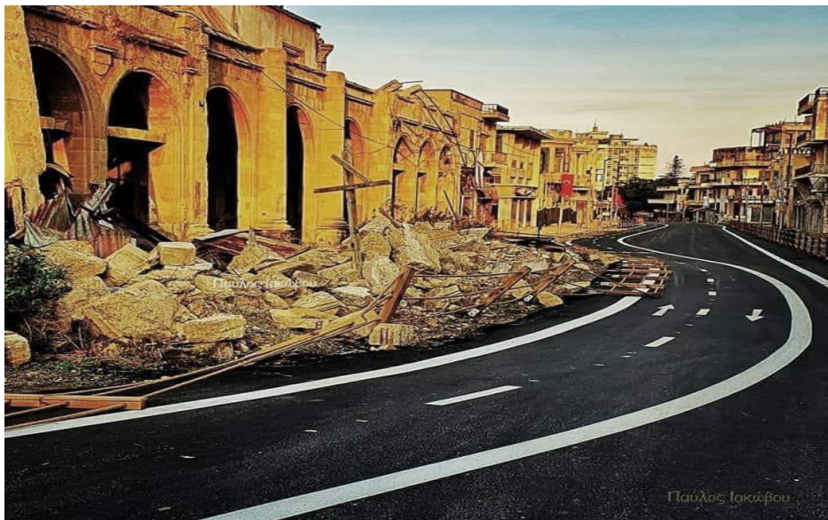
Figure 4.16: The new asphalt by the old Hatjihambi cinema on the Democratias Street. Photo: Pavlos Iacovou – Facebook page circulation
