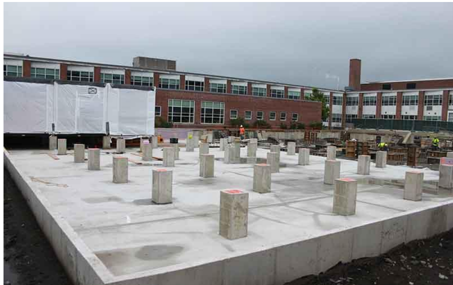
Figure 42: Foundation work for a modular building project (URL37)
