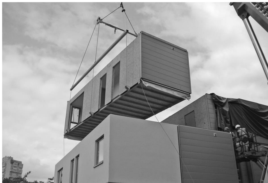
Figure 37: Illustration of open sided modular unit (URL41)
