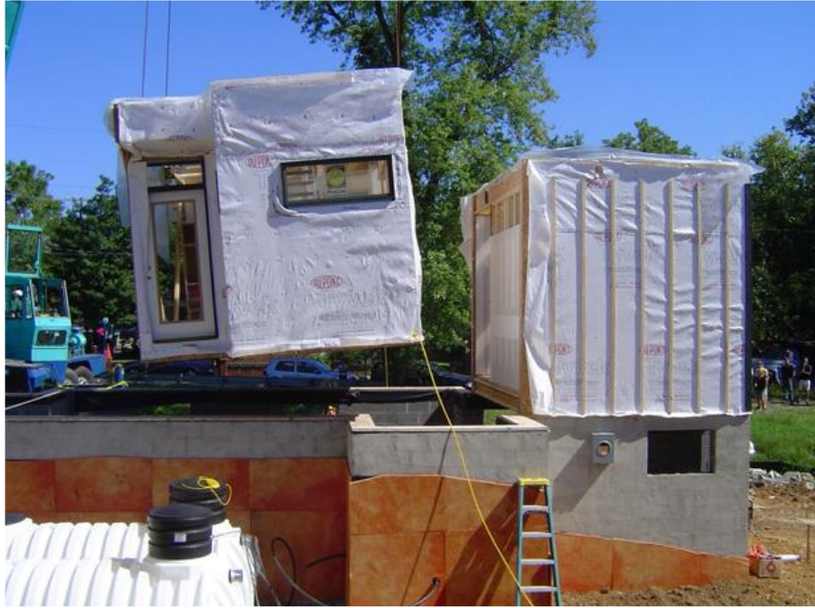
Figure 65: One of the eight modules being placed on the foundation (URL 58)
