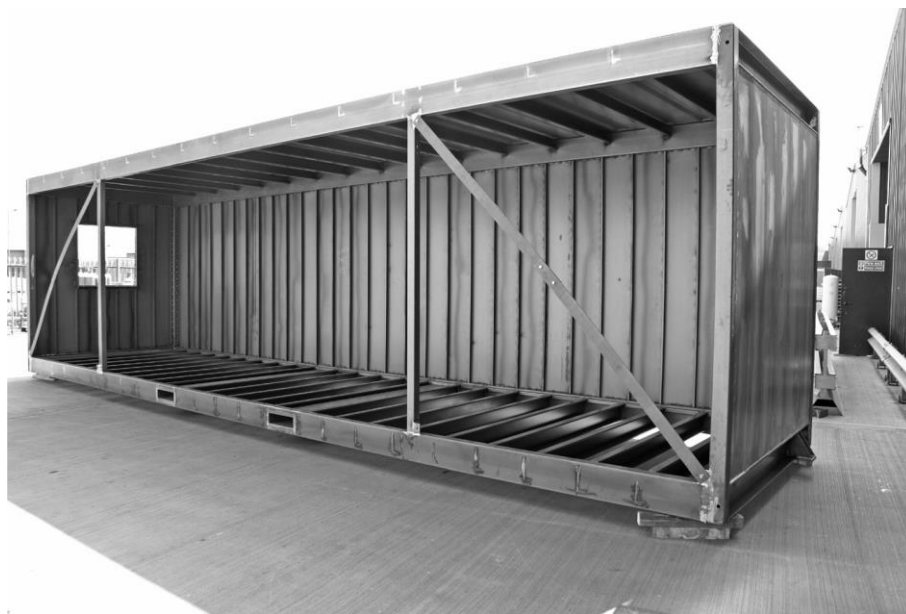
Figure 39: Corner supported module . (URL43)
