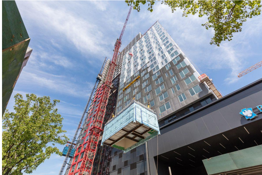
Figure 55: Placing the modules on top of each other (URL52)
