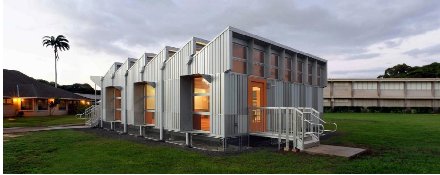
Figure 26: Energy Positive Relocatable Classroom, USA (URL26)
