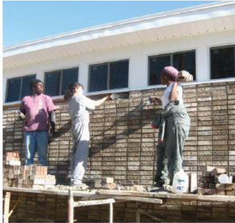
Figure 81: ecoMOD2 team working on façade installation (URL57)
