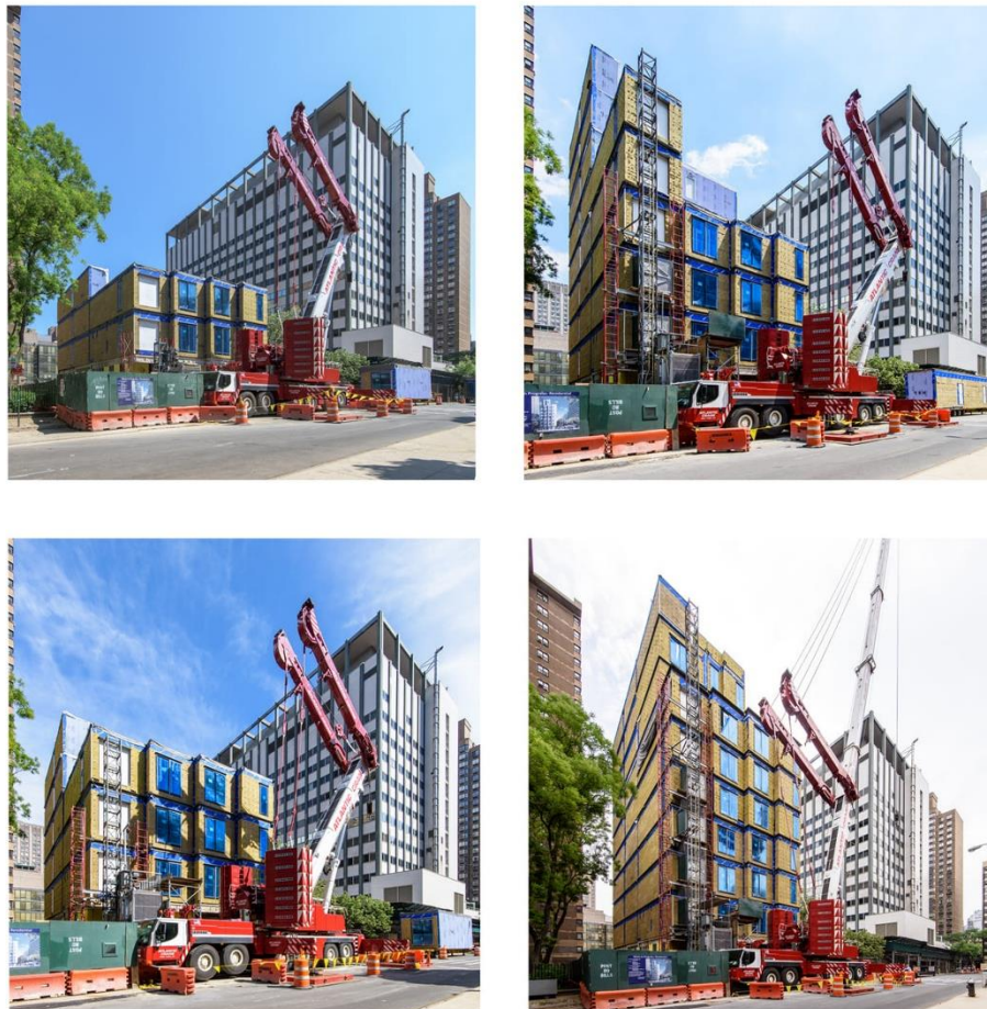
Figure 59: Assembling and installation of the modules on-site (URL56)
