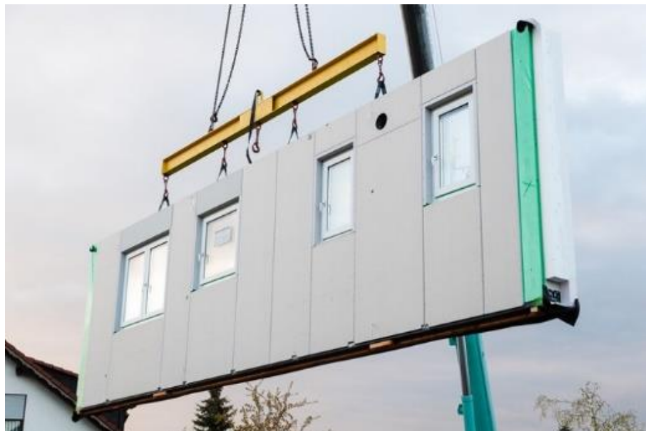
Figure 19: Panellised system. (URL19)
