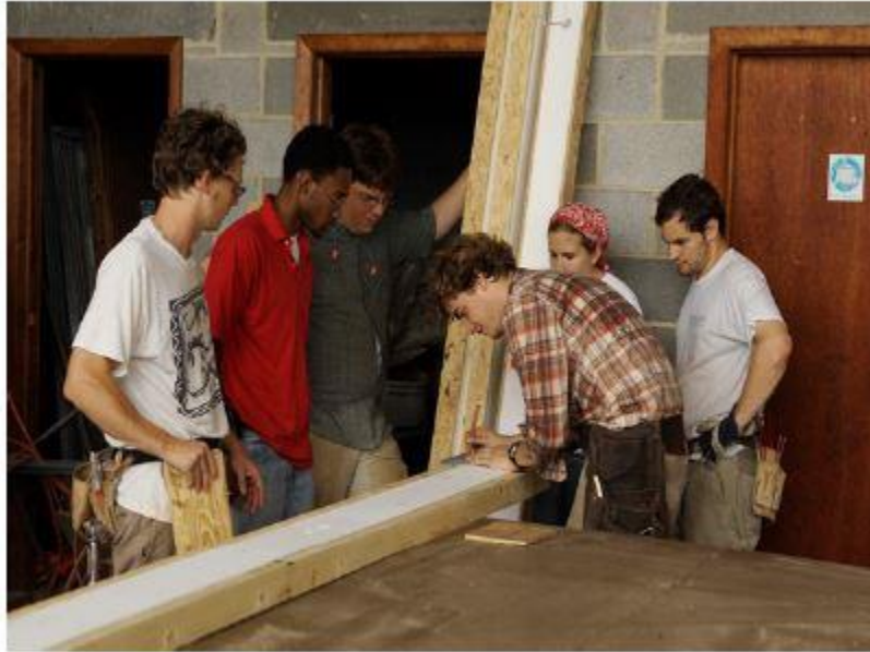
Figure 66: Construction team preparing the modules (URL58)
