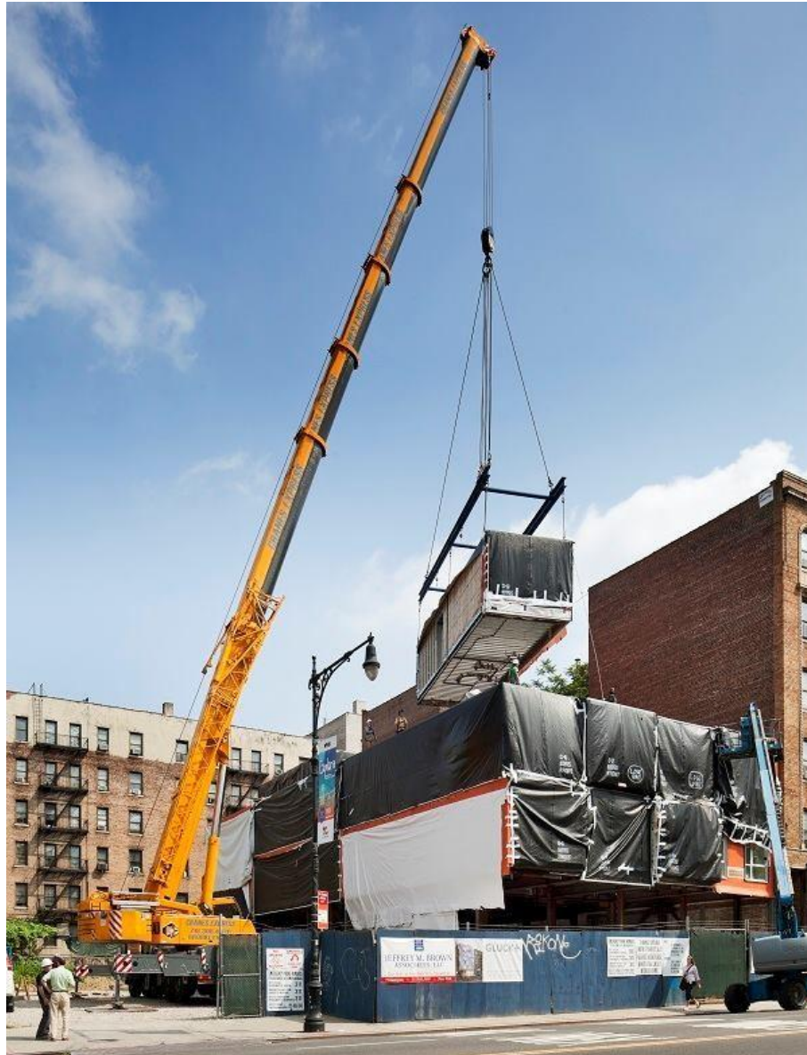
Figure 60: Modules being assembled on the site using a single crane (URL56)
