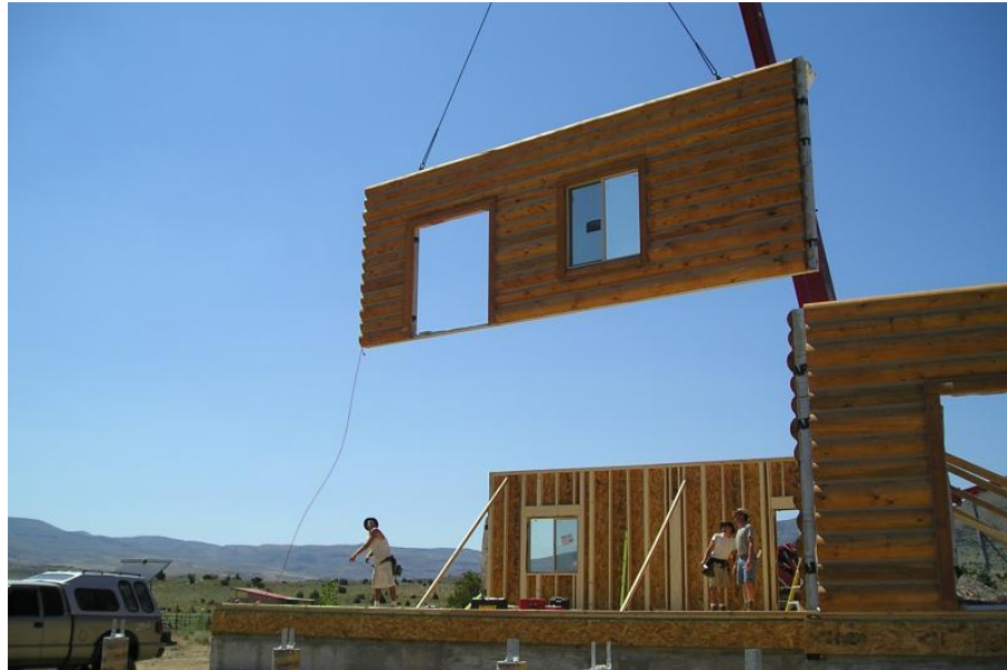
Figure 18: Panelized kit house during assembling process . (URL18)
