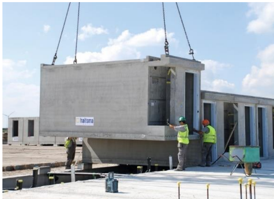
Figure 34: Illustration of a concrete module (URL34)
