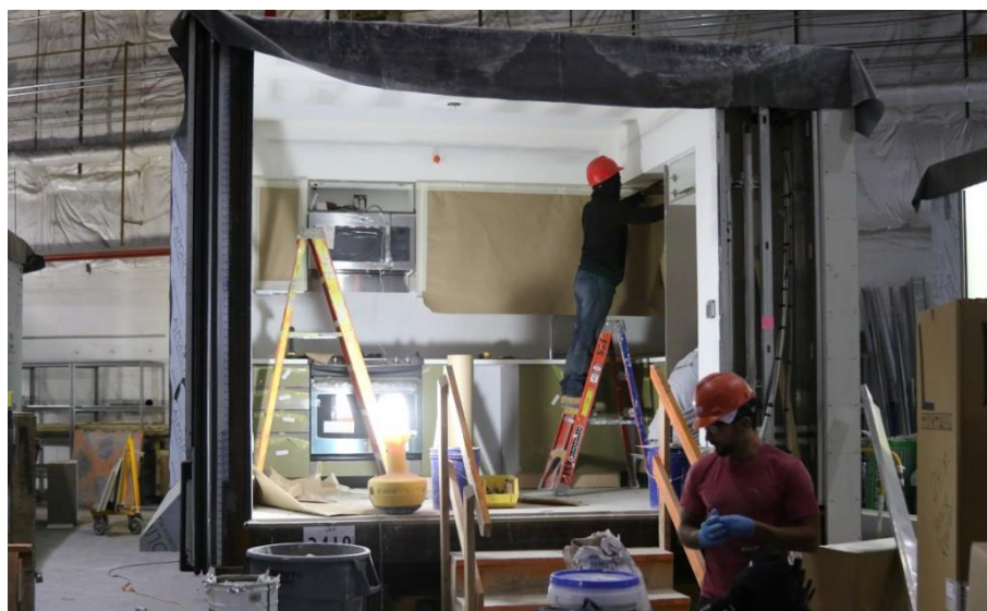
Figure 71: 461Dean module being assembled and prepared in the factory (URL 45)
