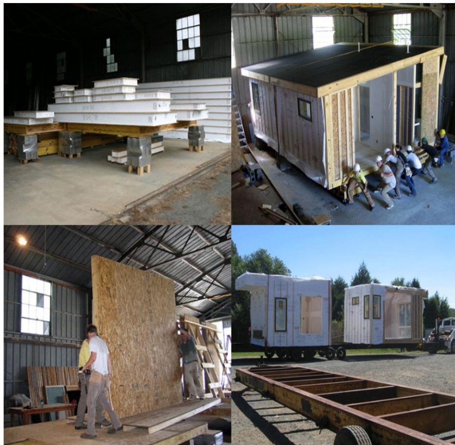
Figure 67: Construction and assembly process (URL 57)
