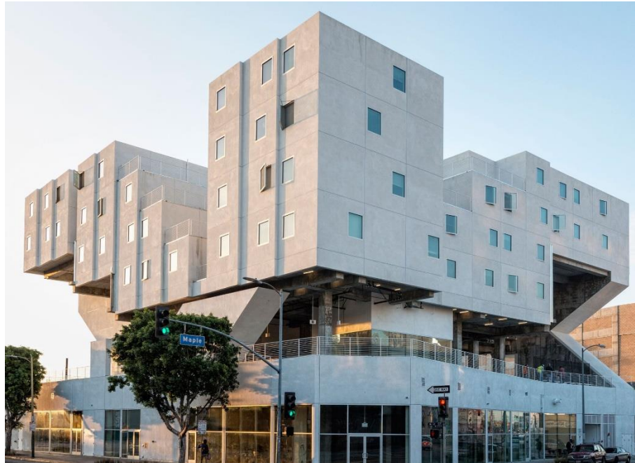
Figure 27: Star Apartments, Los Angeles (URL27)
