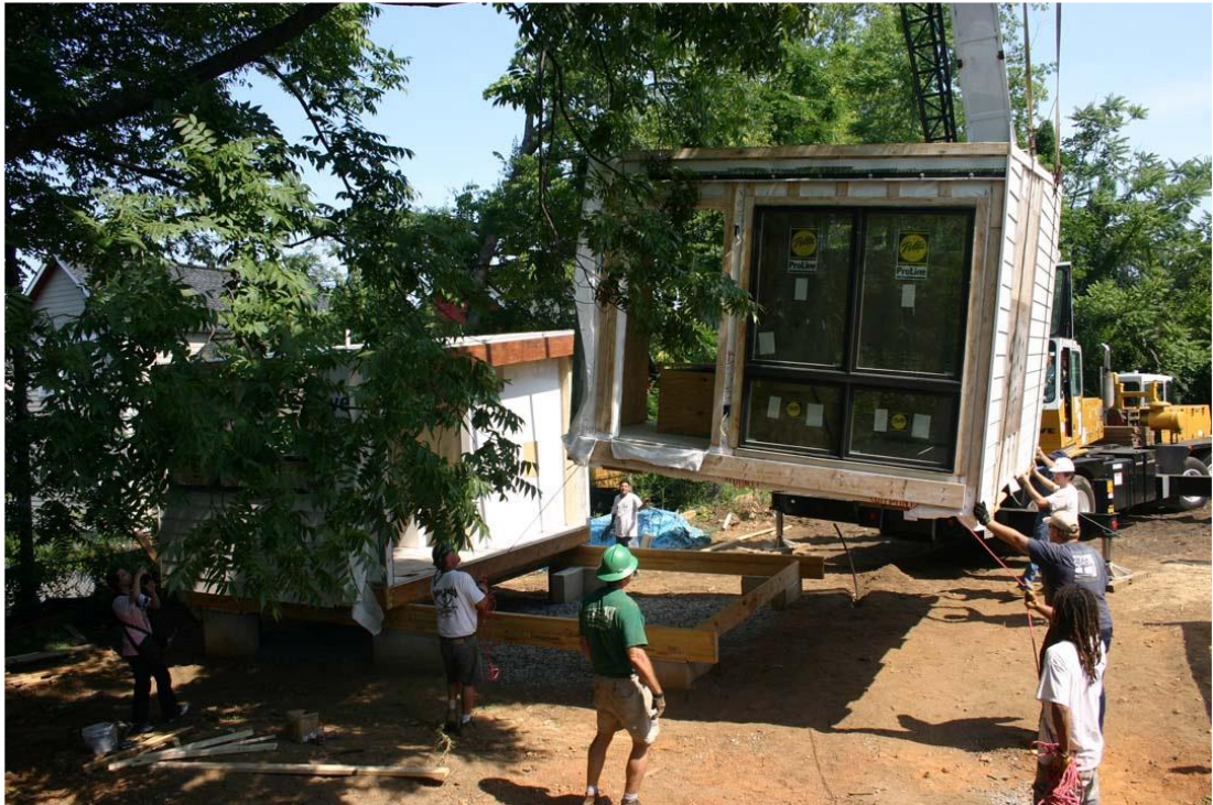
Figure 70: Placing one of the modules of ecoMOD3 on site (URL 58)
