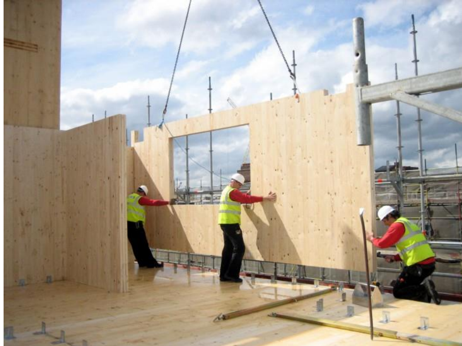
Figure 16: Cross Laminated Timber panel (URL16)
