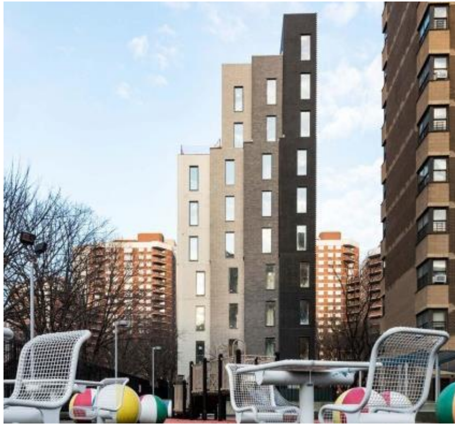
Figure 74: The colors used for the exterior look of the building (URL 47)
