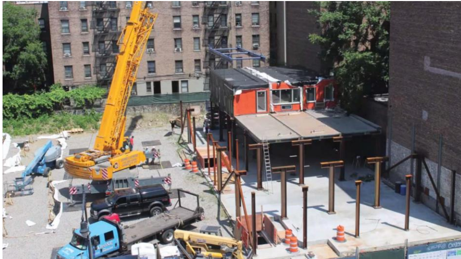
Figure 61: Ground level steel "tree columns" (URL56)
