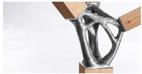
Figure 25: 3D Printed Steel Structure Joints (URL 20)
