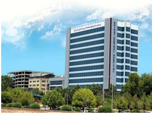
Figure 64. Shiraz Central Hospital Retrieved September 14, 2017, from URL 8.
