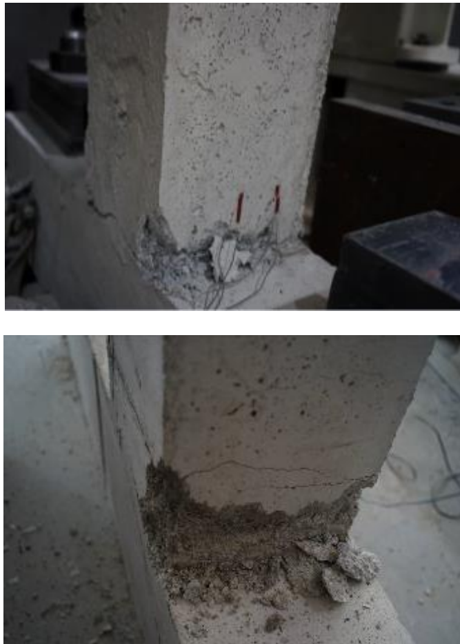
Figure 3.9. Failure of the specimen # 1
