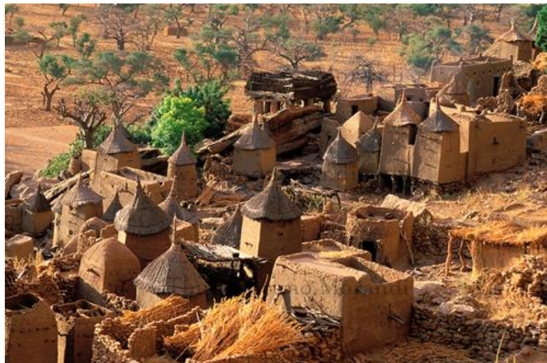
Figure 16: Dogon Structures Built on Cliffs
