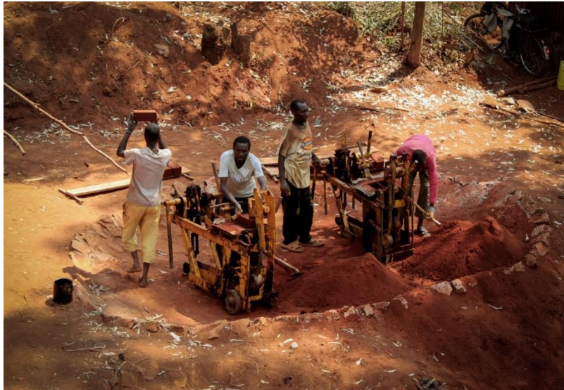
Figure 26: Earth Bricks on Site ("Library of Muyinga / BC Architects," 2020)
