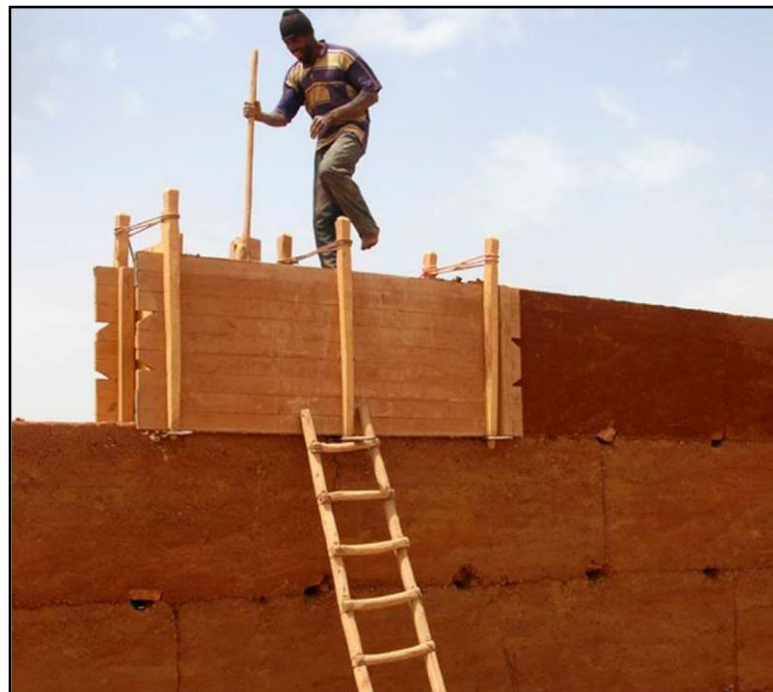
Figure 8: Rammed Earth Construction Walls
