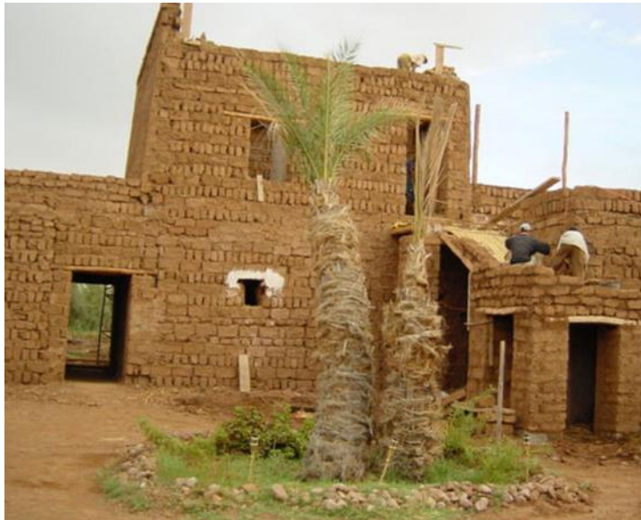
Figure 17: Mud Brick Construction in Da Zarraba Morocco
