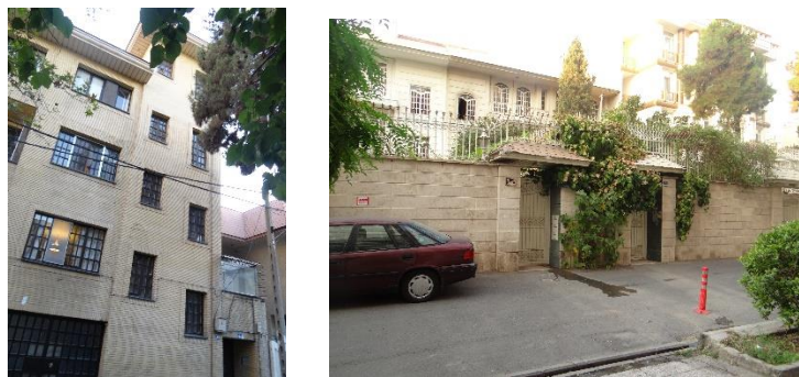
Figure 4.32: Use of marble stone and brick in façade in Tehran case studies (author)
