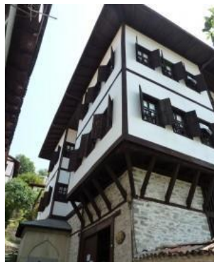
Figure 3.26: Windows' Shutters in Ottoman House, Cyprus (URL10).
