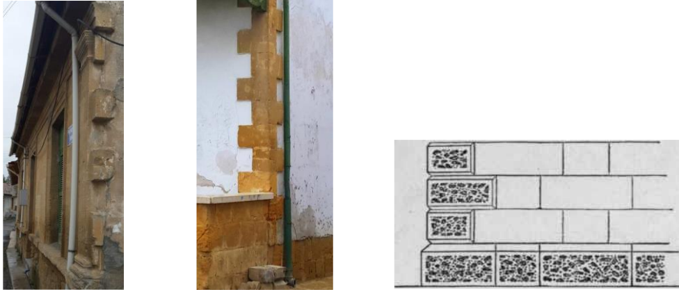
Figure 3.32: Exposed Bond Stone at the Corner (Hafizoglu, 2000; 63).
