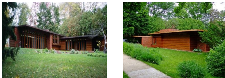
Figure 2.18: Use of wood, Frank Lloyd Wright, Jacobs House, Modison, Wisconsin, 1936, corner details with planet box (shrivastava, 2012; 137).
