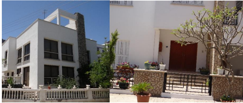
4.55: Use of stone in façade, Famagusta (author).
