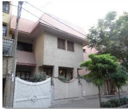
Figure 4.31: Concrete façade in Tehran (author, 2017).
