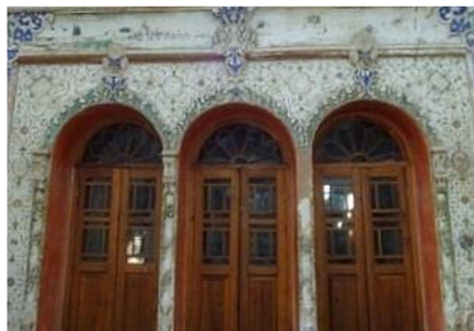
Figure 3.10: Se Dari (three door room) of an Iranian traditional house in Kashan; Iran; (Iran / Iranian Historical Photographs Gallery, 2010; kashan 28).
