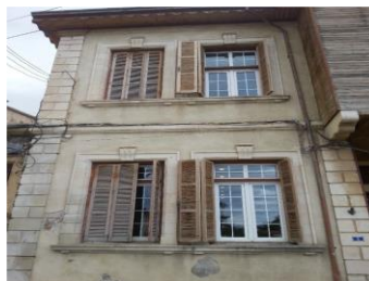
Figure 3.37: Vertical Windows with Timber Shutters (Walled-City, Famagusta), (Dasteri, 2014; 86).
