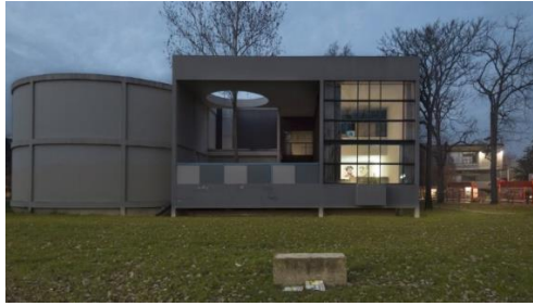
Figure 2.3: Transparency as vertical levels of space; L'Esprit Nouveau Pavilion, by Le Corbusier, Collègè, Paris, France, 1925 (URL2).
