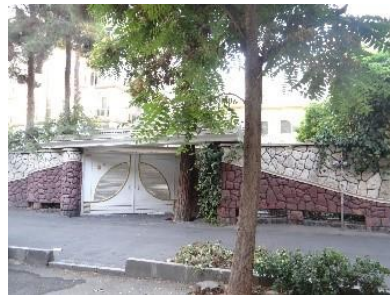
Figure 4.15: Reconstructed detached (author 2017)
