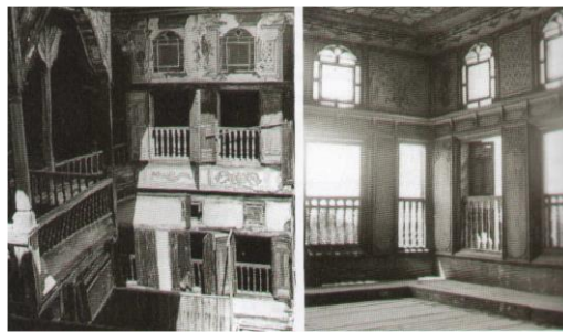
Figure 3.23: The Room Windows (Uluegin, 1998).
