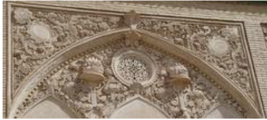
Figure 3.7: Stucco work in Iranian traditional house, Kashan, Iran (Iran / Iranian Historical Photographs Gallery, 2010; kashan 29).
