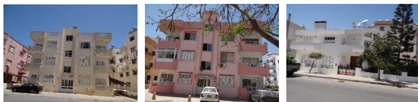
Figure 4.47: Utilizing shutter in front of windows, Famagusta (author)
