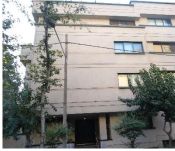
Figure4.27: Horizontal line in façade in Tehran example (author, 2017).
