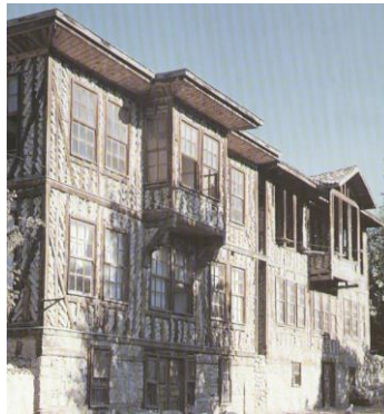
Figure 3.30: Baghdadi Construction System (Ahunbay, & Aksoy, 2005)
