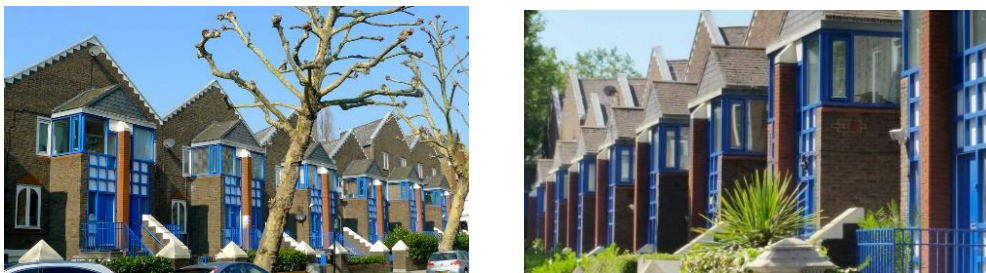
Figure 2.63: St. Mark's Road (New London Architecture) ( Gossel, leuthouser, 1971; 249)
