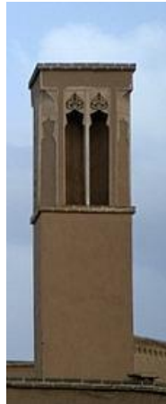
Figure 3.12: Wind catcher of one Iranian traditional house in Kashan, Iran; (Iran / Iranian Historical Photographs Gallery, 2010; kashan 18).
