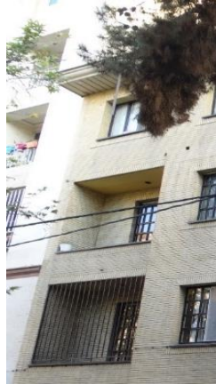
Figure 4.24: Enclosed balcony in Tehran case study (author)
