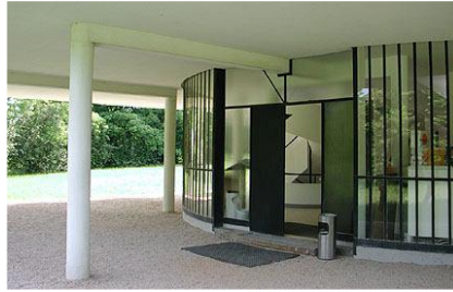
Figure 2.43: Pilotis (supporting columns) (Corbusier, 2001; 134)
