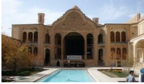
Figure 3.9: Biruni (common part) of an Iranian traditional house in Kashan, Iran; (Iran / Iranian Historical Photographs Gallery, 2010; kashan, 05).
