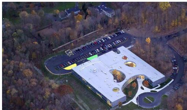
Figure 5: The outside view of Burr Street elementary school
