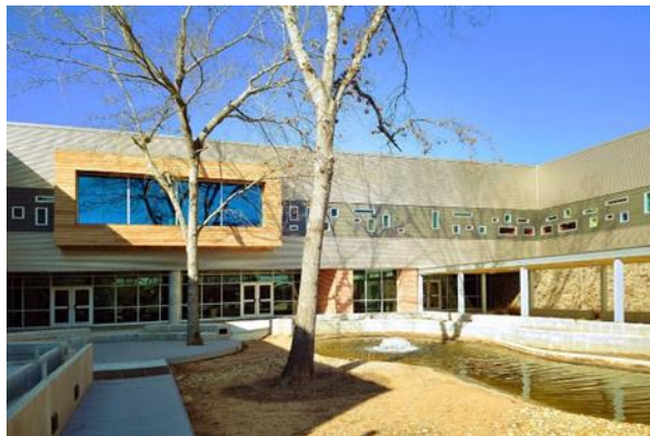
Figure 7: External entrance of Gloria Marshall elementary school
