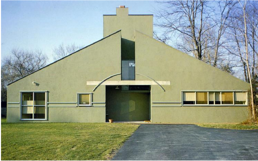
Figure 15: Vanna Venturi House – Composition of primary shapes Robert Venturi – 1964 - United States (URL 4)
